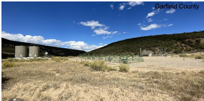
South West corner of location.
