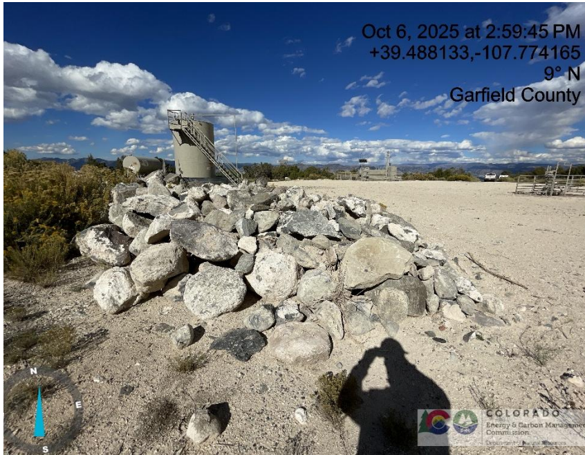
Photo # 4466 Soil stockpile covered in rocks
