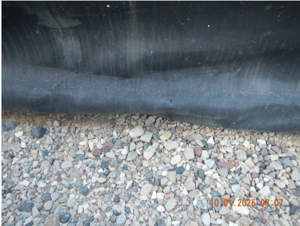
Berm liner has several puncture holes near bottom of berm walls.
