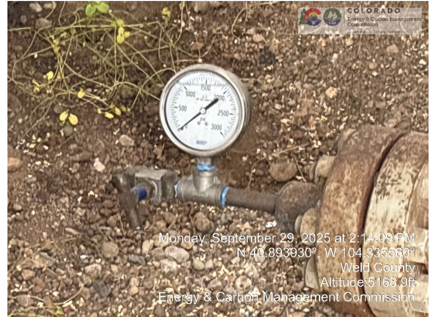
Photo 4 – Casing Gauge
