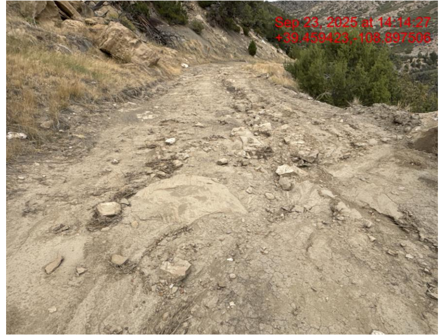
Erosion of Lease Road – Photo #00898
