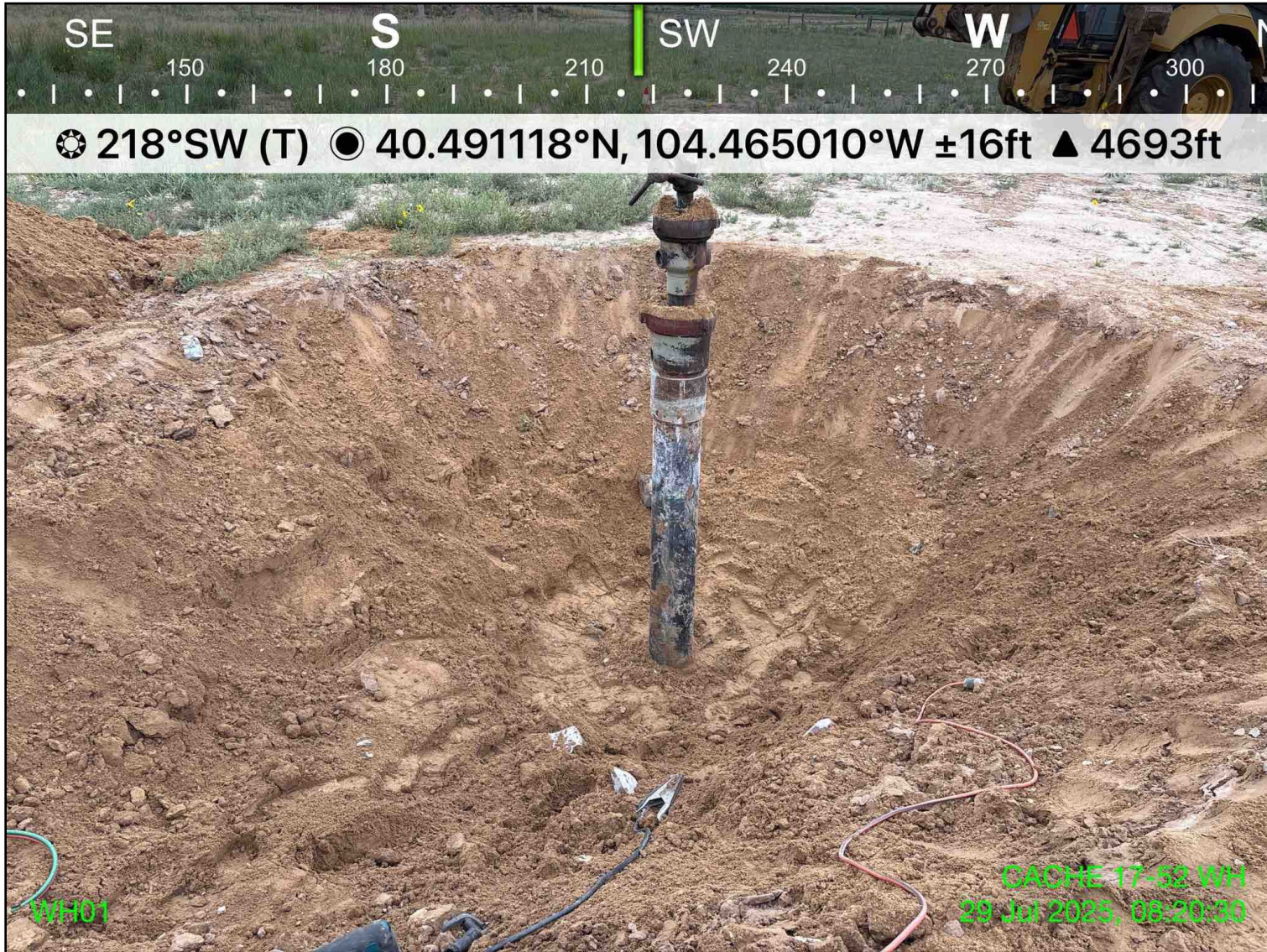
Photo 4: View of WH01 sample location and excavation, facing southwest
