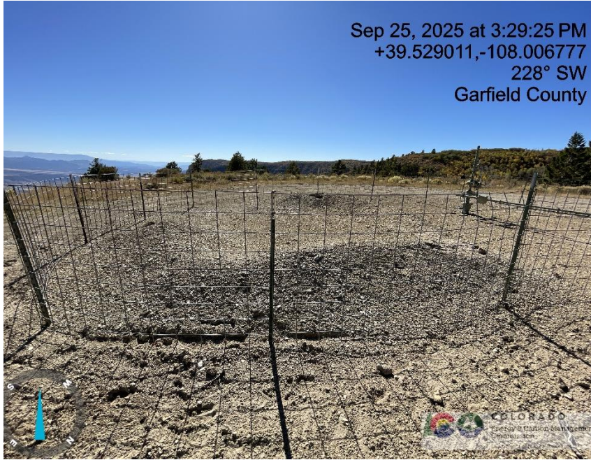
Photo # 3211 Soil stockpile with no BMP's
