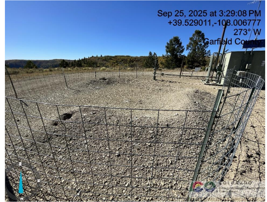
Photo # 3212 Soil stockpile with no BMP's
