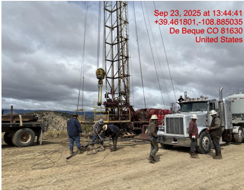
Plugging Ops – Photo #00882
