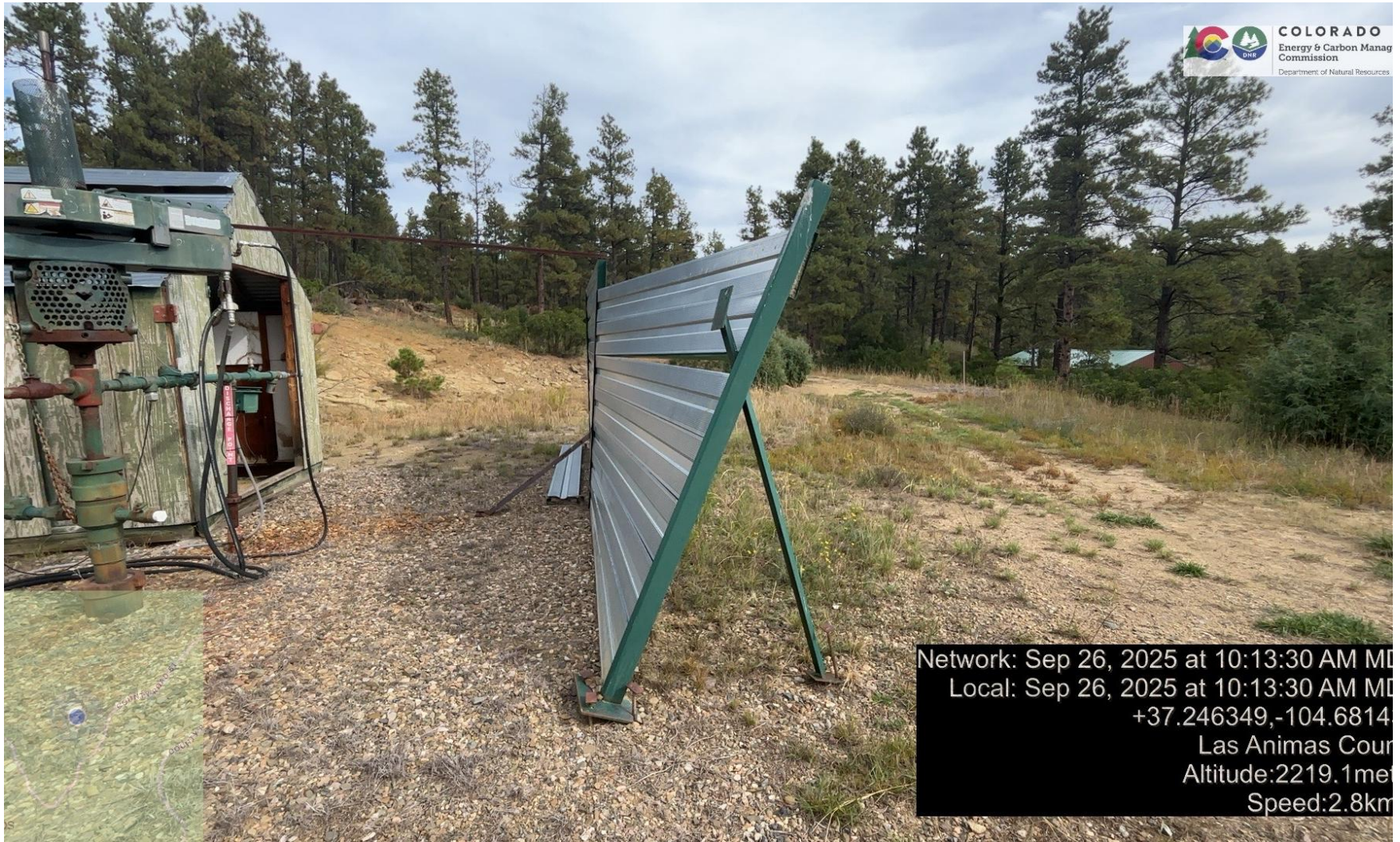
PHOTO 3: SOUND WALLS ARE IN DISREPAIR. REPAIR SOUNDWALLS. CA DATE 10-26-2025.
