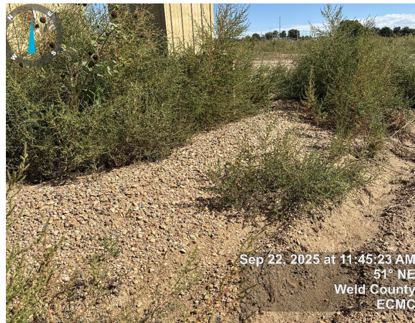
Photo 8: berm not maintained
