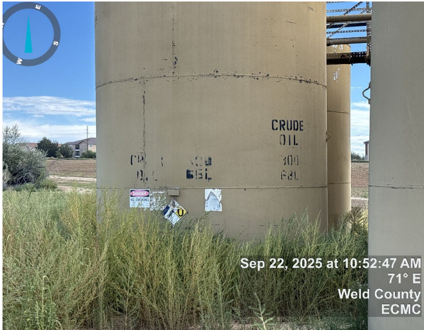
Photo 15: NFPA placard damaged
