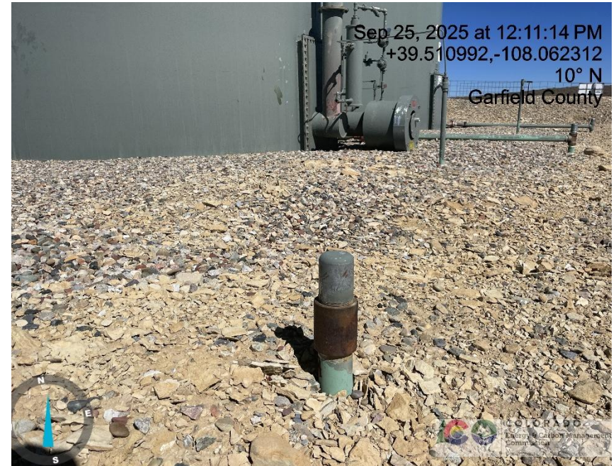
Photo # 2529 Unused flowline lacks lockout tagout (OOSLAT)
