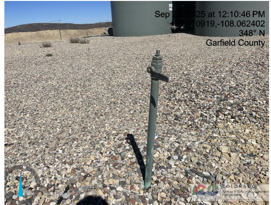
Photo # 2527 Unused flowline lacks lockout tagout (OOSLAT)
