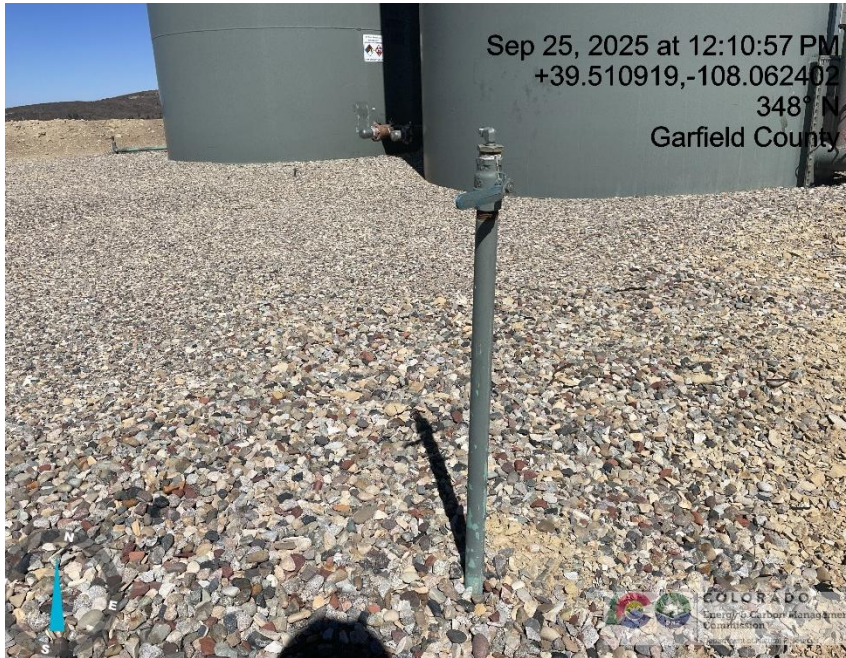
Photo # 2528 Unused flowline lacks lockout tagout (OOSLAT)
