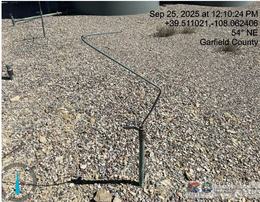
Photo # 2526 Unused flowline lacks lockout tagout (OOSLAT)
