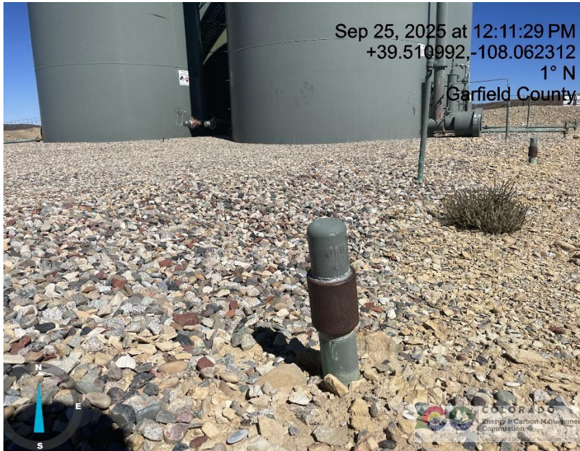
Photo # 2530 Unused flowline lacks lockout tagout (OOSLAT)
