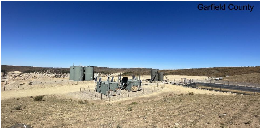
South West corner of location.
