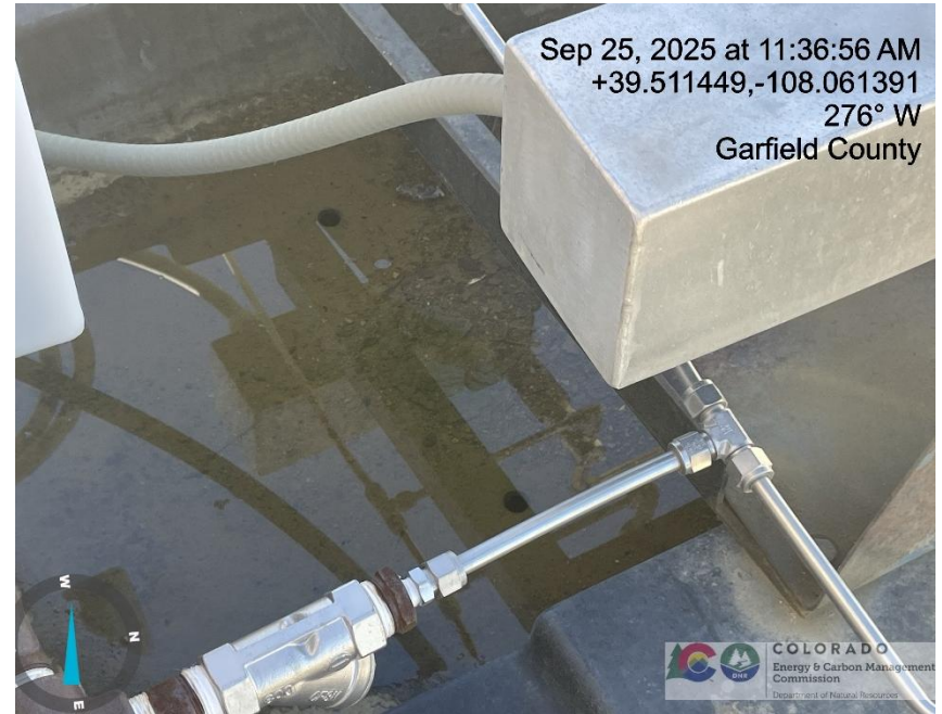
Photo # 2551 Failure to maintain chemical BMP – Chemical tank containment approximately 3/4 full of fluid/BMP insufficient to contain possible spill (Additionally standing fluid on containment constitutes a wildlife hazard)
