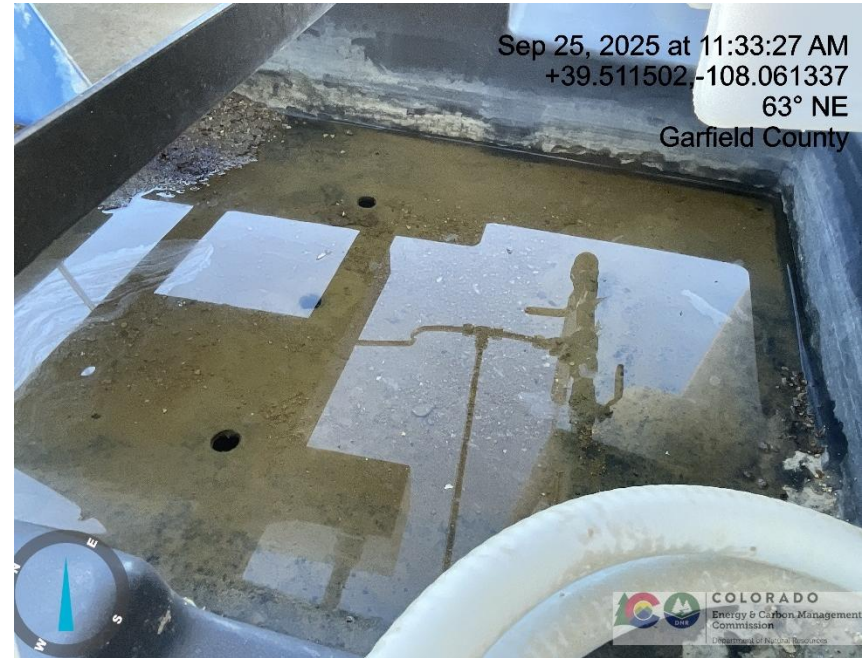
Photo # 2549 Failure to maintain chemical BMP – Chemical tank containment approximately 3/4 full of fluid/BMP insufficient to contain possible spill (Additionally standing fluid on containment constitutes a wildlife hazard)
