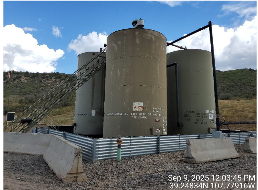
Tank Battery with metal berm
