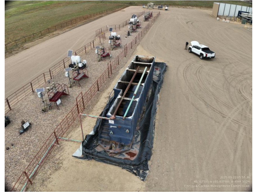
Missing Bird protector on tank
