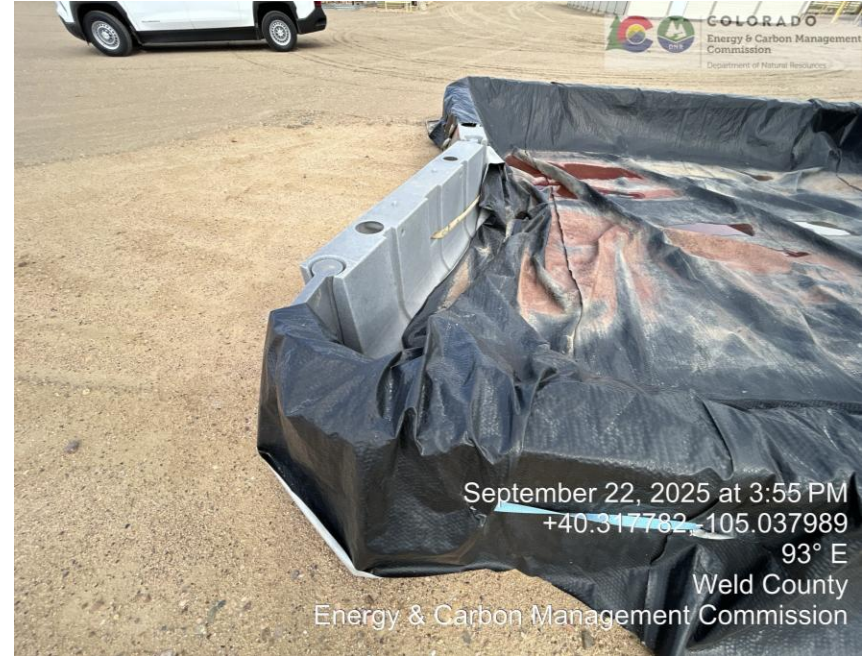
Liner needs fixed or replaced
