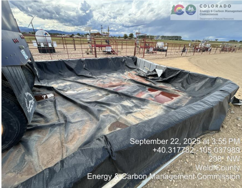
Rain water in secondary containment
