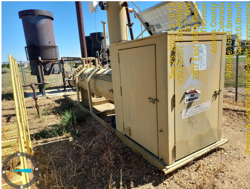
Photo 7 Horizontal Heated Separator.
