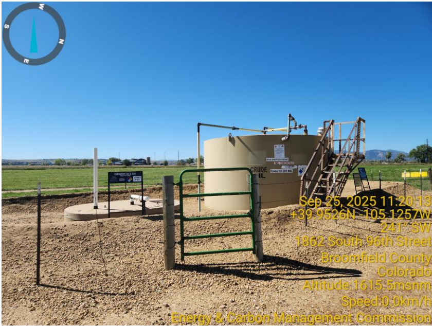
Photo 3 Tank Battery.
