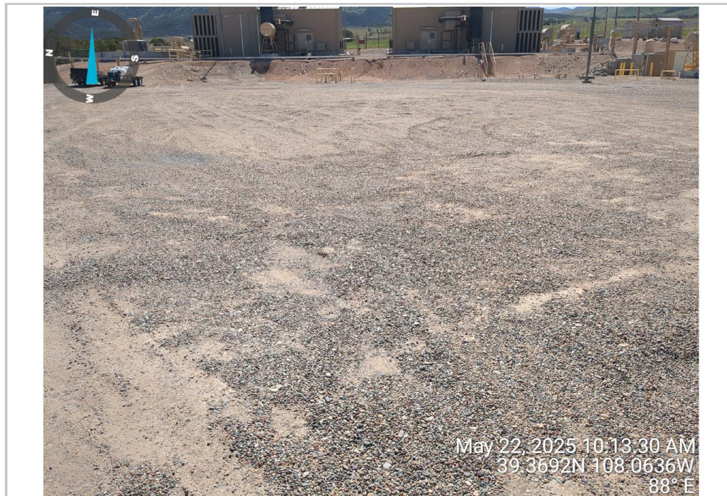
Former Well Pad - Western Perimeter, Facing East
