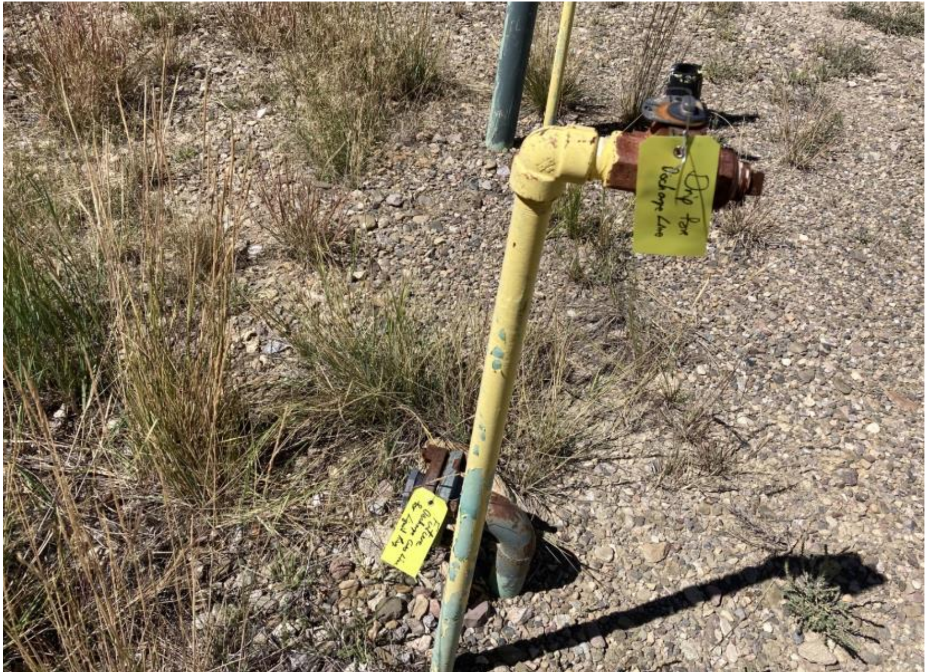
PHOTO 2: ALL RISERS HAVE BEEN LABELED AND IDENTIFIED.
