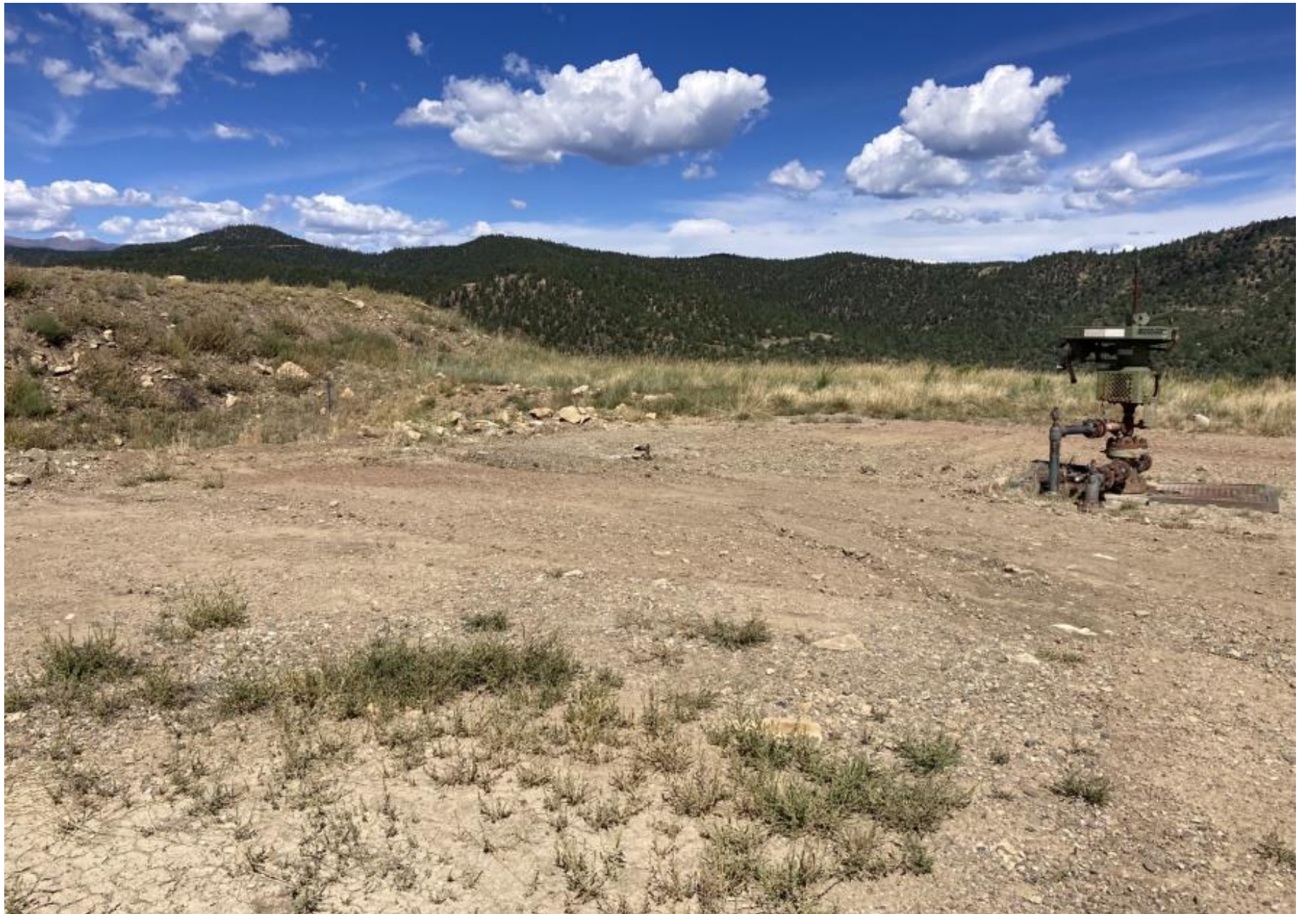
PHOTO 1: THE SOIL STAINS HAVE BEEN REMOVED FROM LOCATION AND ALL OPERATING EQUIPMENT HAS RECEIVED MECHANICAL INSPECTION. THE UNUSED ENGINE SKID AND SOUNDWALLS HAVE ALSO BEEN REMOVED.
