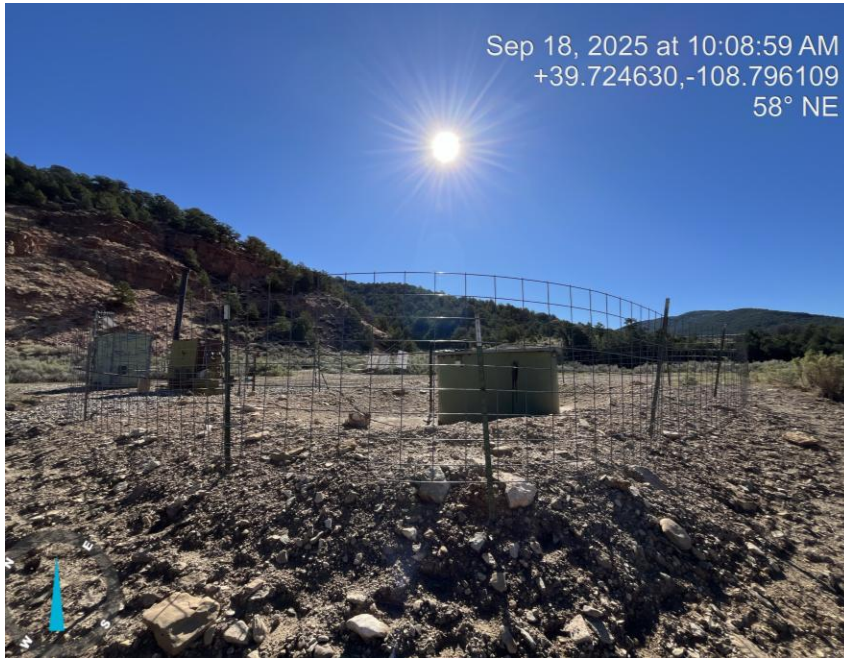
Photo # 3614 NW corner of location
