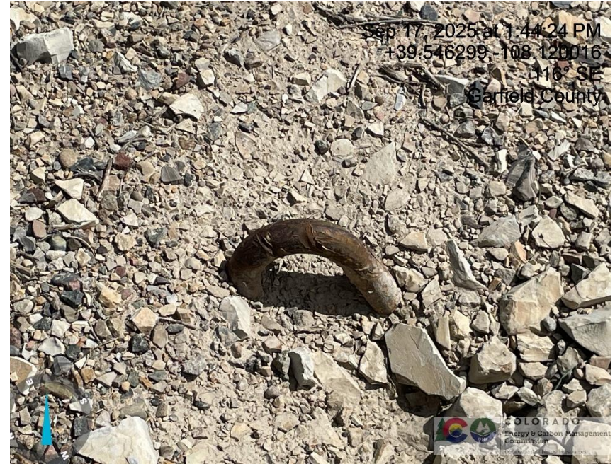
Photo # 707 Unmarked deadman
