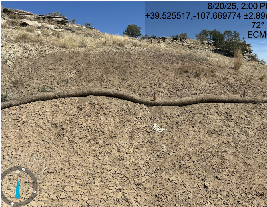
Erosion on cut slope and BMP's failing
