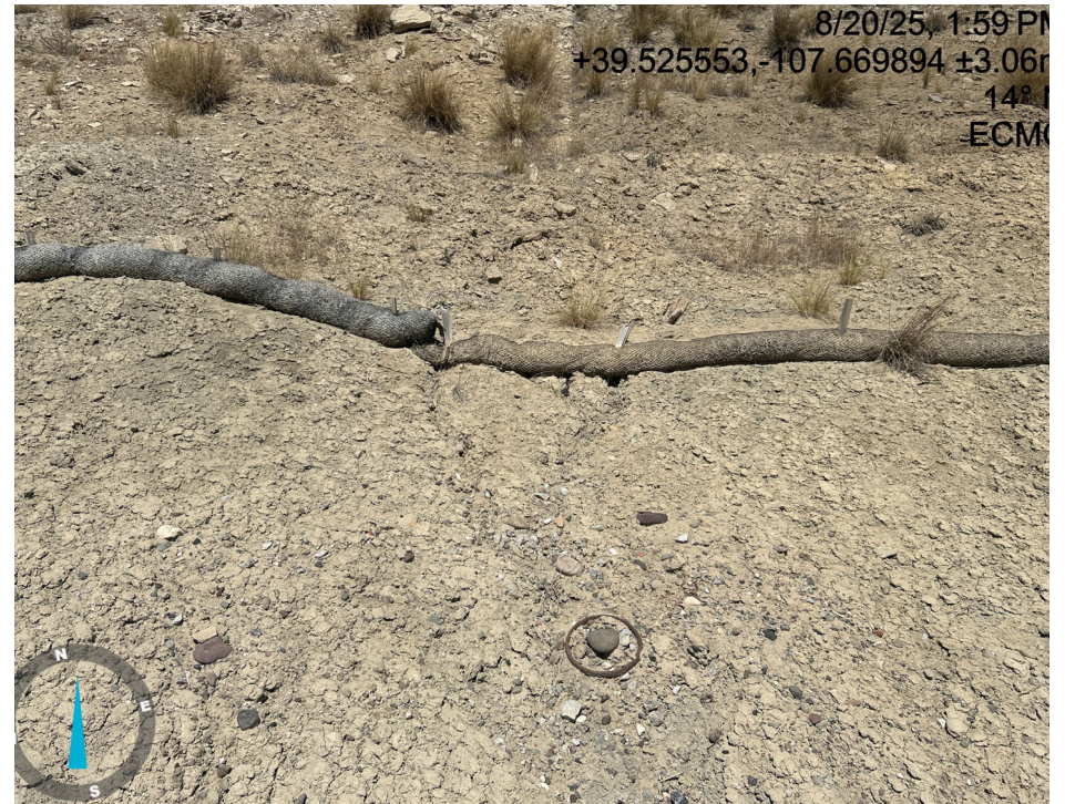
Erosion on cut slope and BMP's failing
