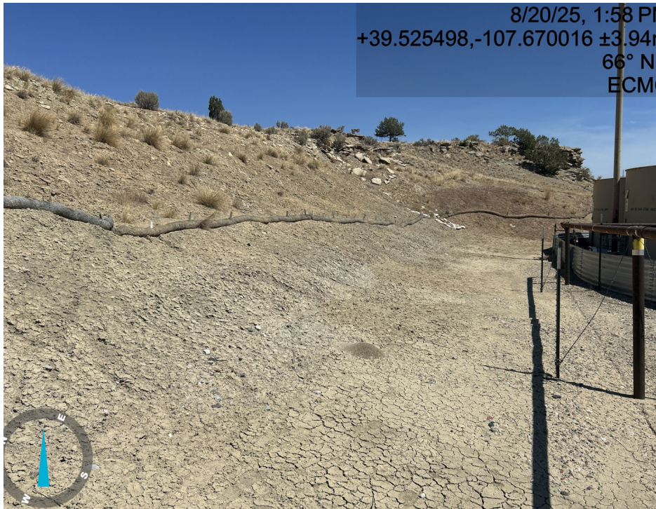
Erosion on cut slope and BMP's failing
