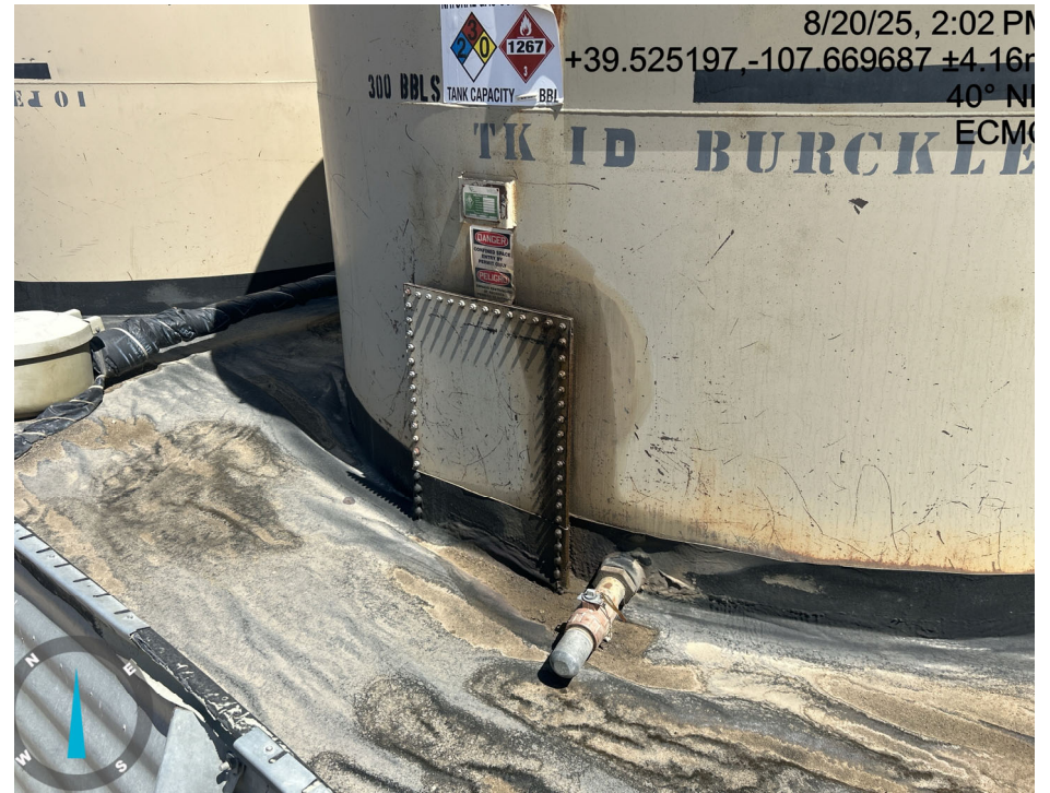
Man way leaking?
