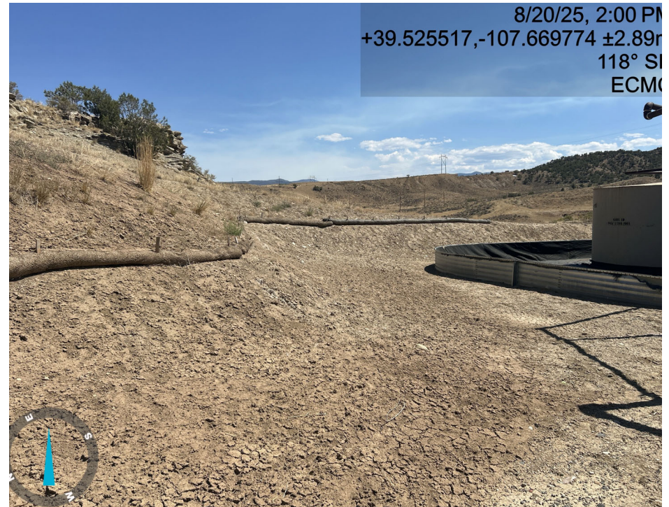
Erosion on cut slope and BMP's failing
