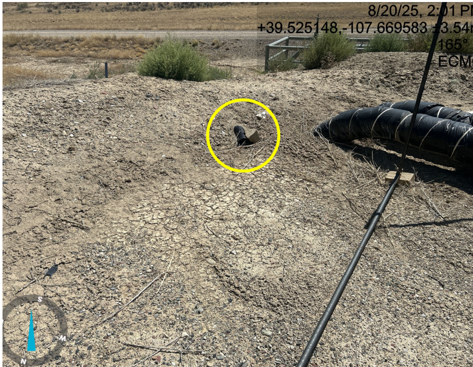
Drain line from location
