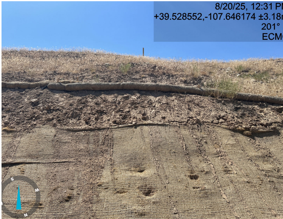
Cut slope erosion
