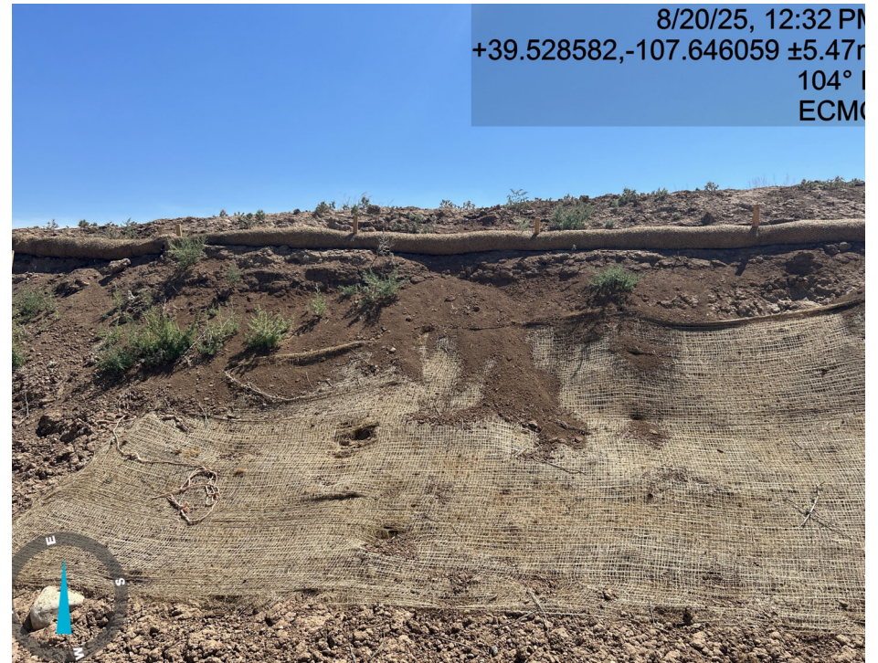
Cut slope erosion
