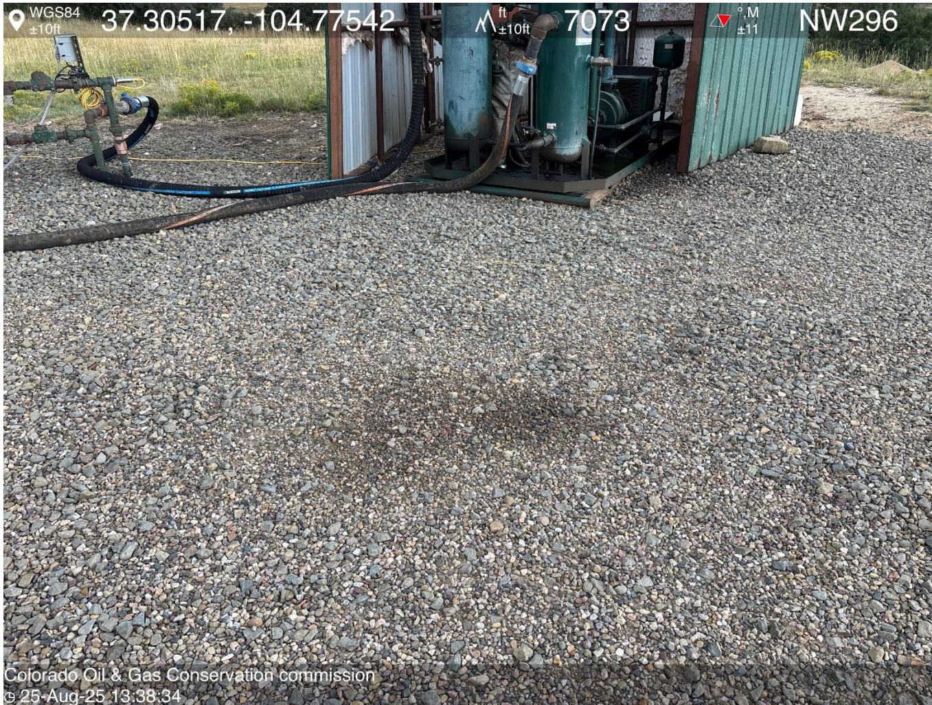
PHOTO 5: AREA OF IMPACTED SOIL NEAR COMPRESSOR SKID. Conduct maintenance on equipment, cleanup stained material and review self inspection processes. COMPLY WITH RULE 1002,(2).D. CA DATE 9-25-2025.
