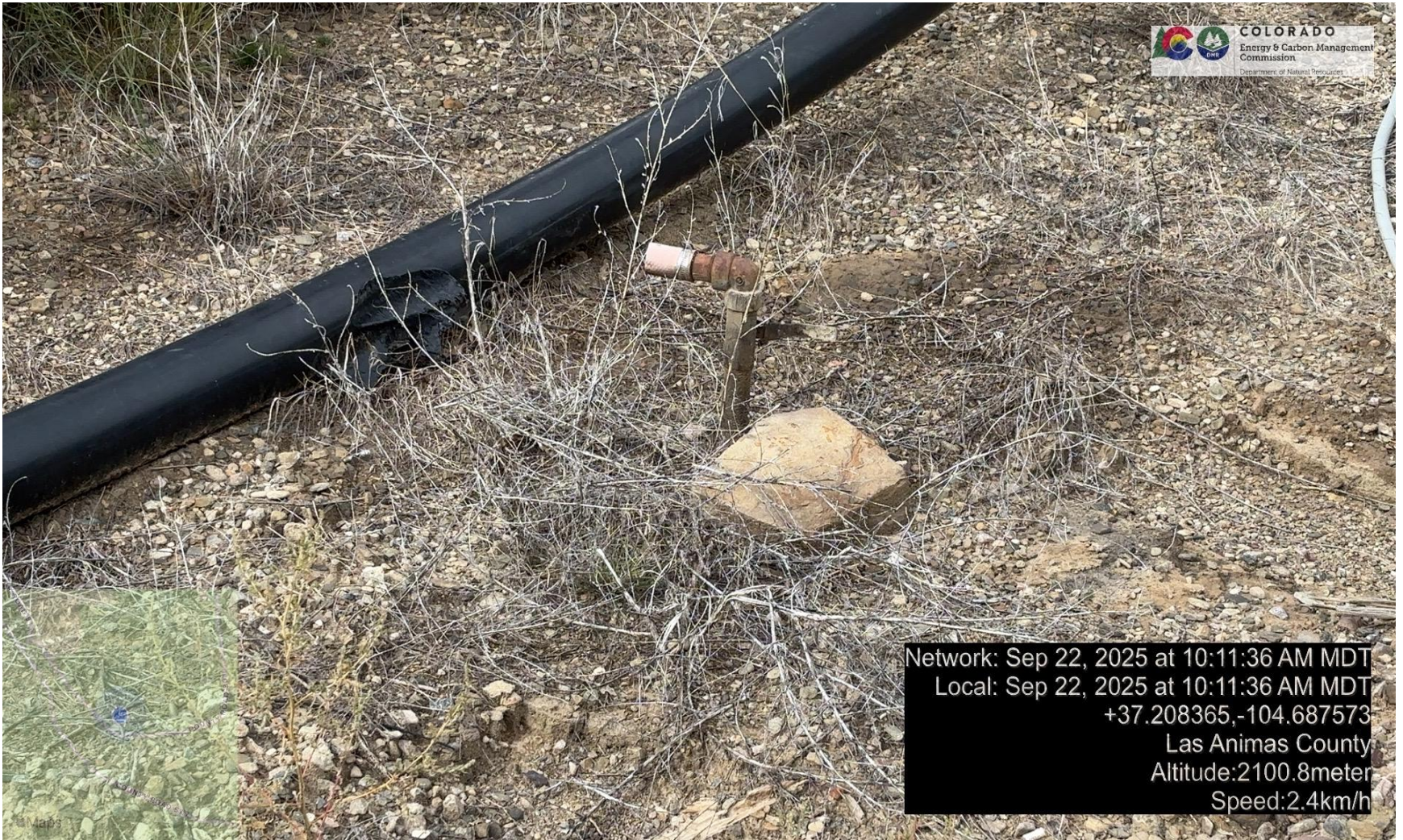
PHOTO 3: UNUSED 1" RISER NEAR PUMPJACK. USE REMOVE OR MARK UNUSED RISER PER RULE 606. CA DATE 10-22-2025.
