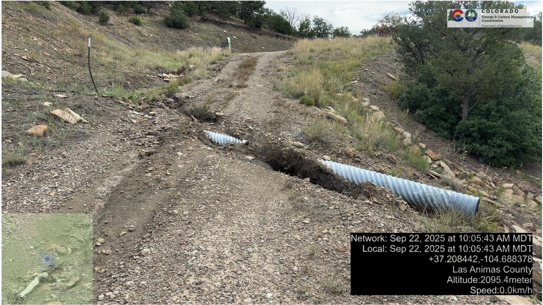
PHOTO 5: STORMWATER BYPASSED CULVERT DUE TO CULVERT BEING PLUGGED AND HAS WASHED OUT ROAD. REPAIR ROAD, CLEAN CULVERT AND REPAIR ALL BMP'S ALONG THIS ROW PER RULE 1002. CA DATE 10-22-2025.
