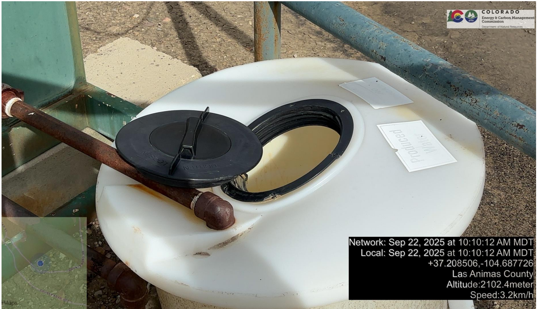
PHOTO 4: TANK LID MUST REMAIN INSTALLED OR SOME OTHER FORM OF WILDLIKE PROTECTION NEEDS TO BE IN PLACE.
