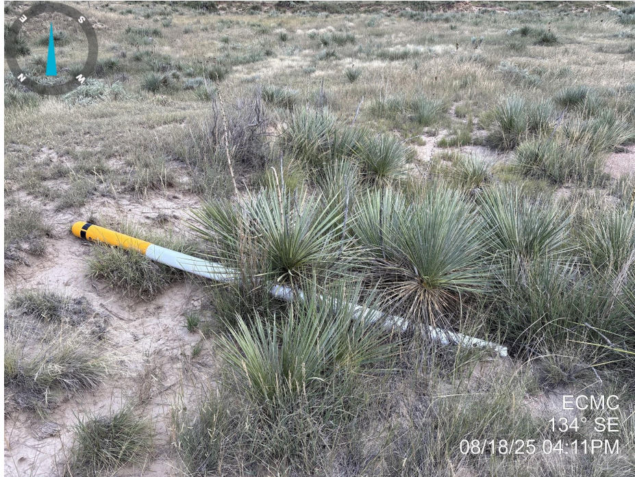
Photo 7. Photo taken from the access road, facing southeast. Photo illustrates midstream equipment that has fallen over.
