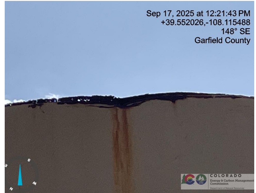
Photo # 278 Tank failure/tank lacks integrity
