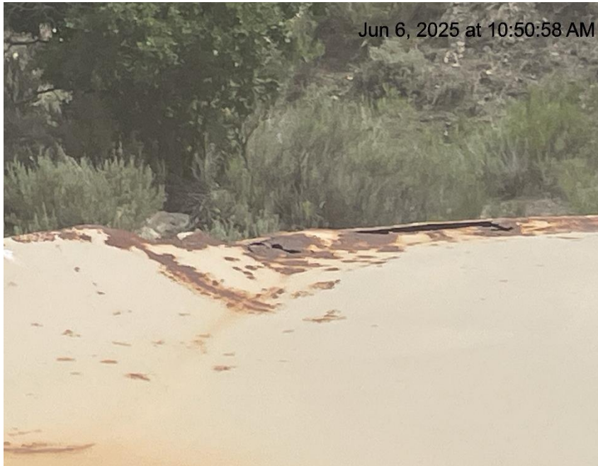
Photo # 6901 From inspection/audit 708906677 conducted on 06/06/2025 Tank failure Multiple holes in tank/tank lacks integrity
