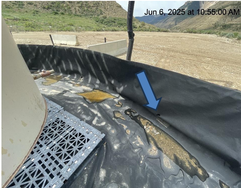
Photo # 6915 From inspection/audit 708906677 conducted on 06/06/2025 Hole in liner/liner needs maintenance
