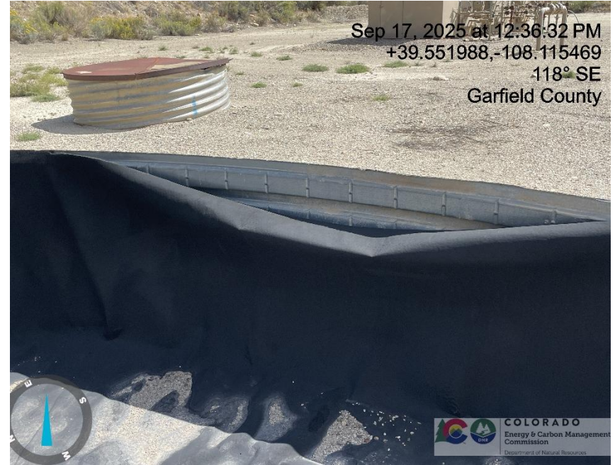
Photo # 286 Liner in disrepair/liner needs maintenance
