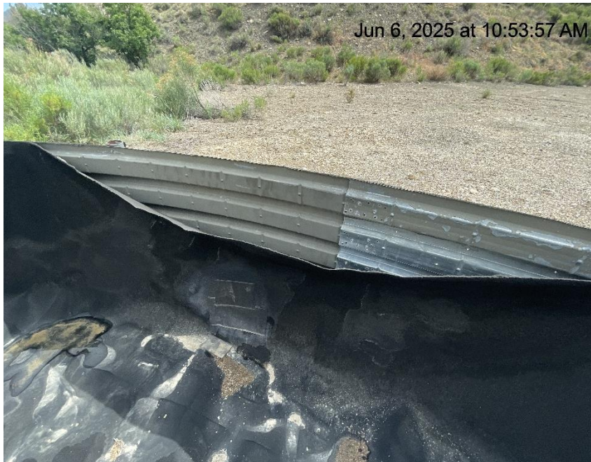
Photo # 6908 From inspection/audit 708906677 conducted on 06/06/2025 Liner in disrepair/liner needs maintenance
