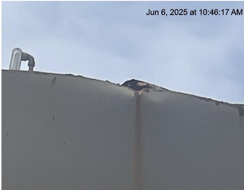
Photo # 6898 From inspection/audit 708906677 conducted on 06/06/2025 Tank failure/tank lacks integrity
