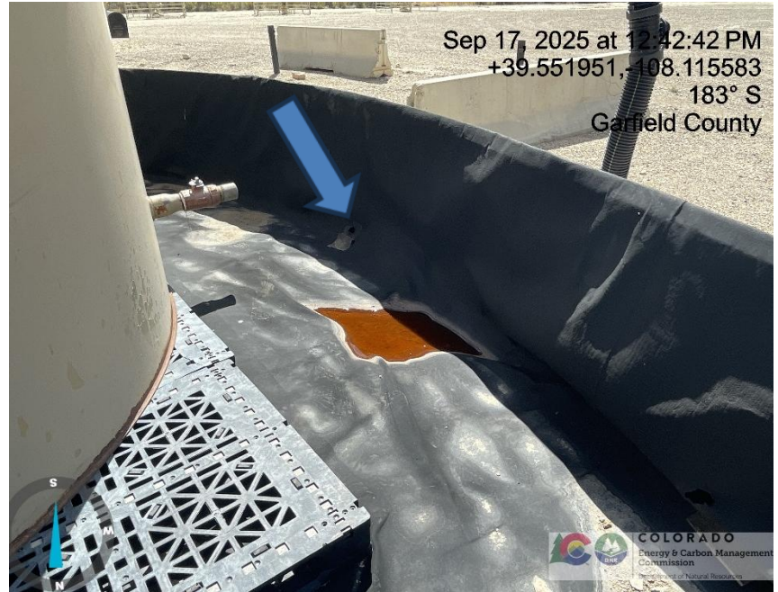
Photo # 293 Hole in liner/liner needs maintenance
