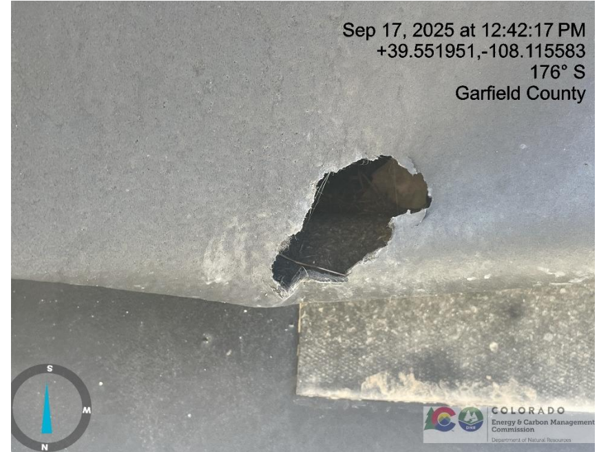
Photo # 292 Hole in liner/liner needs maintenance
