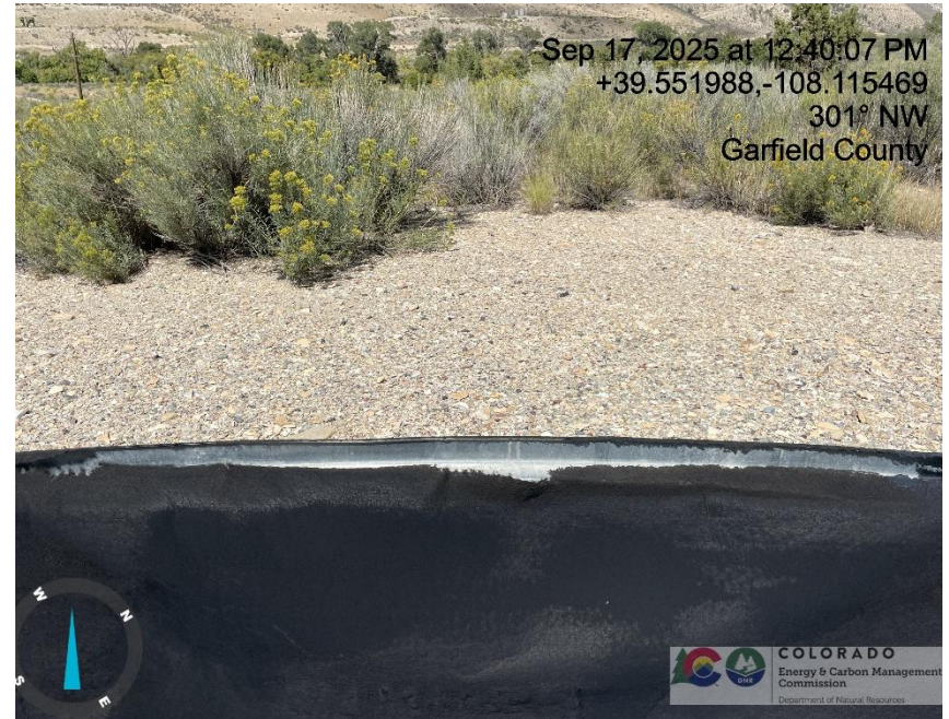
Photo # 295 Liner in disrepair/liner needs maintenance
