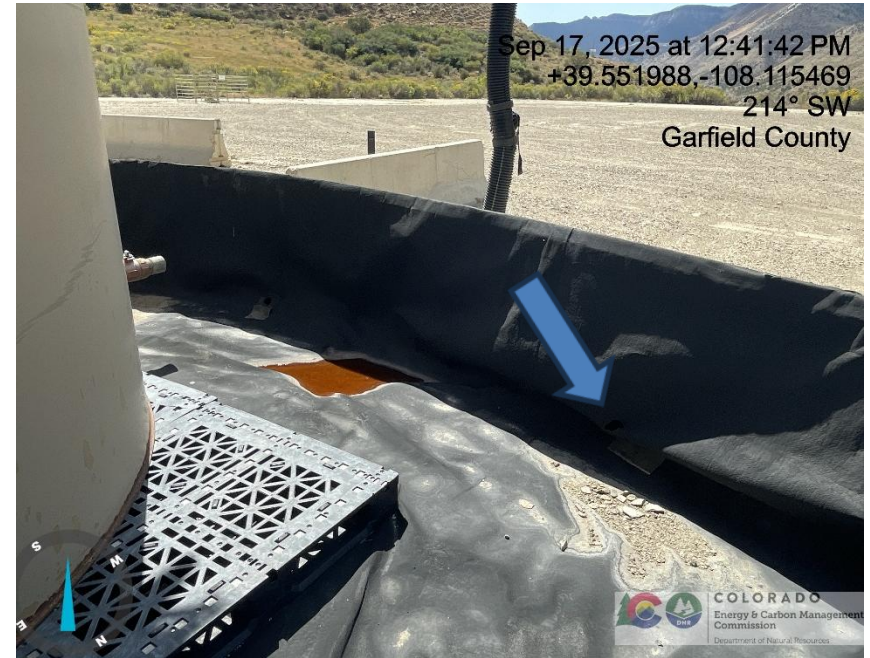
Photo # 291 Hole in liner/liner needs maintenance
