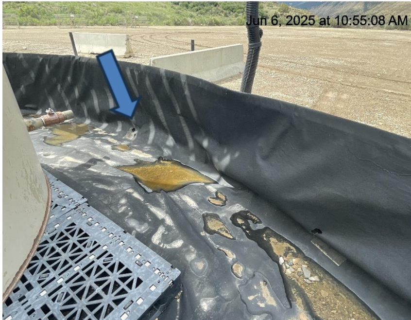
Photo # 6917 From inspection/audit 708906677 conducted on 06/06/2025 Hole in liner/liner needs maintenance
