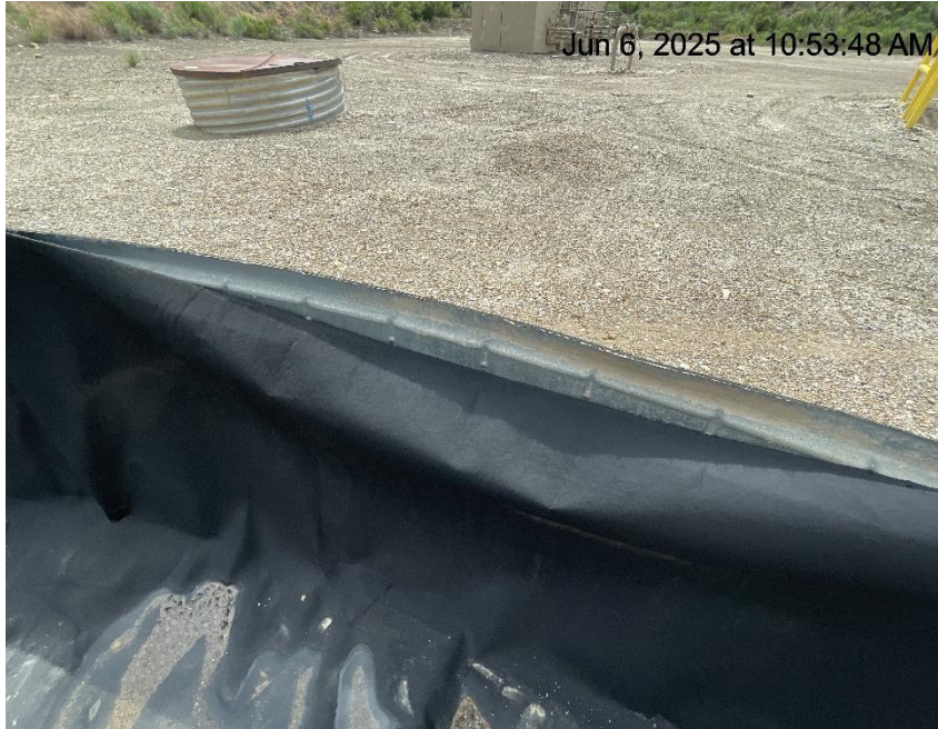
Photo # 6907 From inspection/audit 708906677 conducted on 06/06/2025 Liner in disrepair/liner needs maintenance
