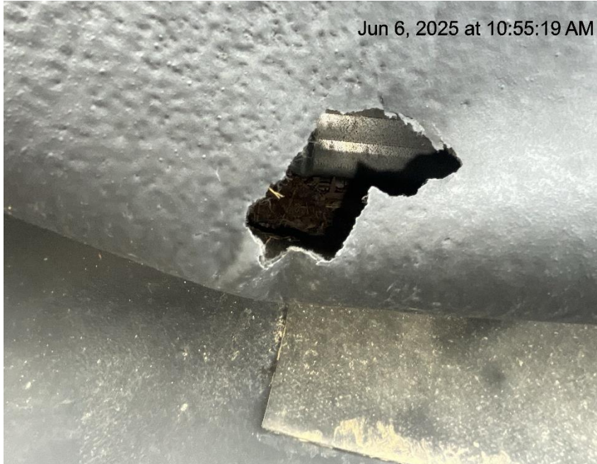
Photo # 6916 From inspection/audit 708906677 conducted on 06/06/2025 Hole in liner/liner needs maintenance
