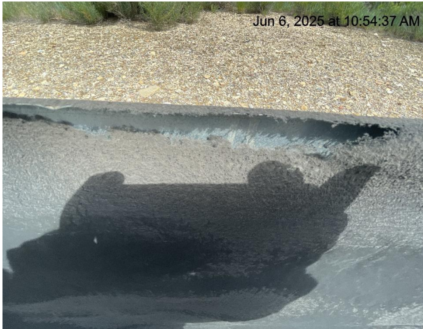
Photo # 6919 From inspection/audit 708906677 conducted on 06/06/2025 Liner in disrepair/liner needs maintenance
