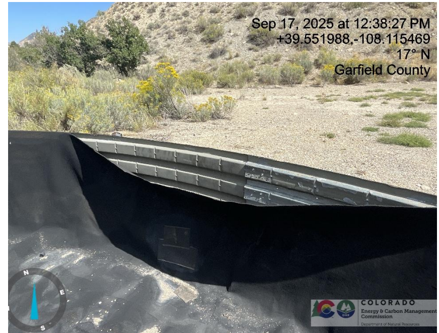
Photo # 287 Liner in disrepair/liner needs maintenance
