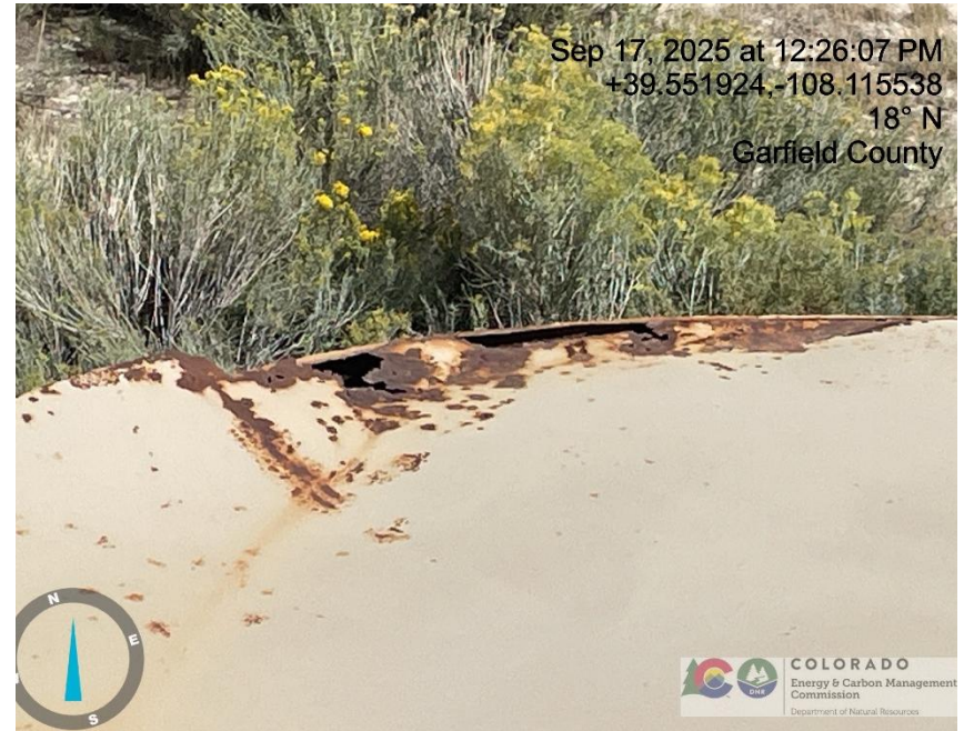
Photo # 280 Tank failure Multiple holes in tank/tank lacks integrity
