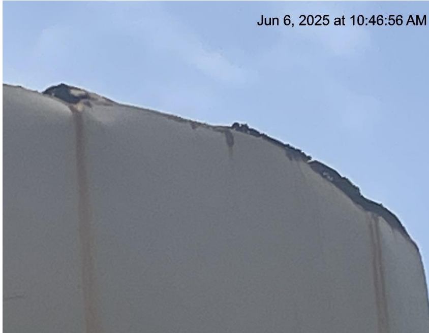
Photo # 6897 From inspection/audit 708906677 conducted on 06/06/2025 Tank failure/tank lacks integrity
