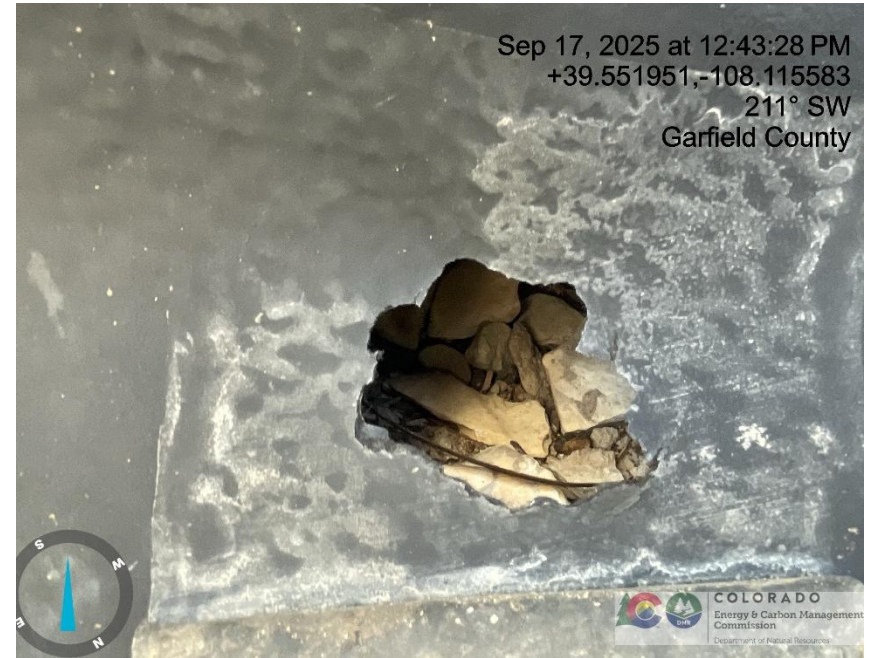
Photo # 294 Hole in liner/liner needs maintenance
