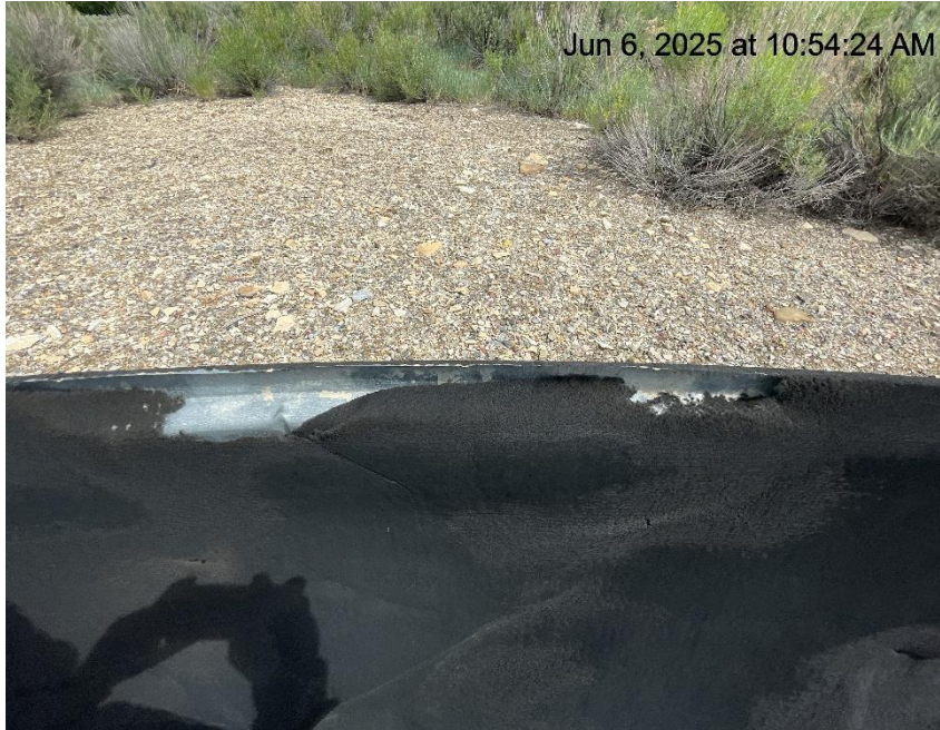
Photo # 6912 From inspection/audit 708906677 conducted on 06/06/2025 Holes in liner/liner needs maintenance
