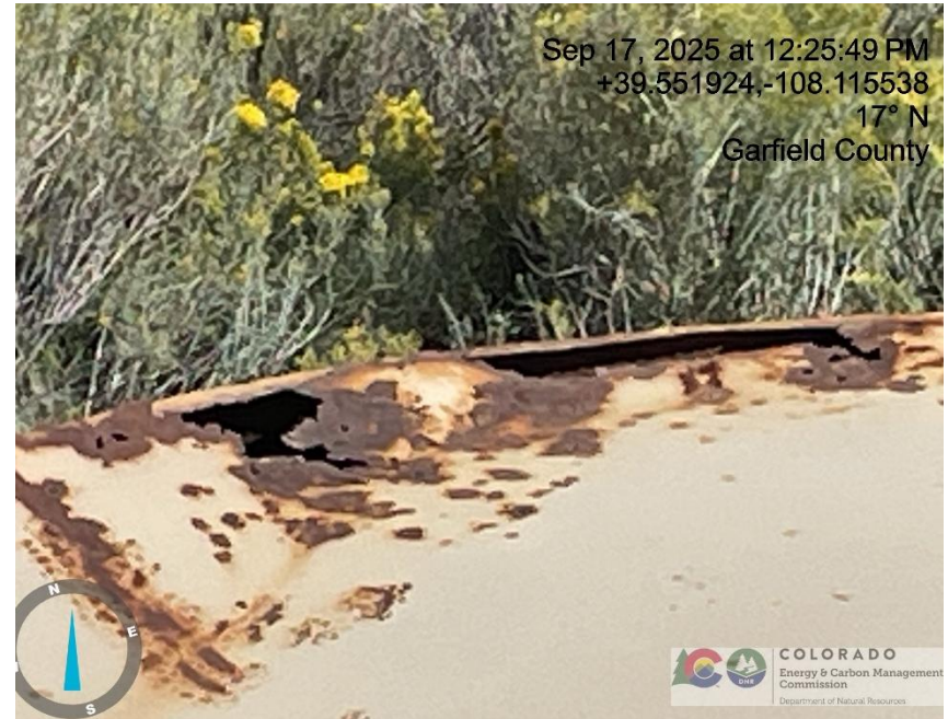
Photo # 279 Tank failure Multiple holes in tank/tank lacks integrity
