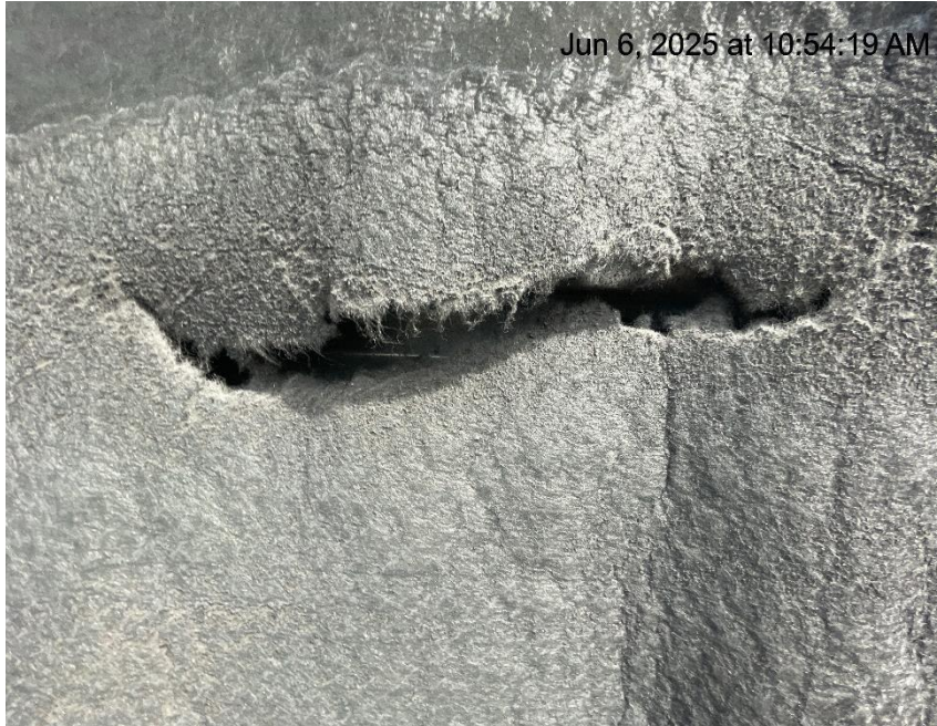
Photo # 6911 From inspection/audit 708906677 conducted on 06/06/2025 Hole in liner/liner needs maintenance
