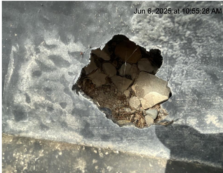
Photo # 6918 From inspection/audit 708906677 conducted on 06/06/2025 Hole in liner/liner needs maintenance
