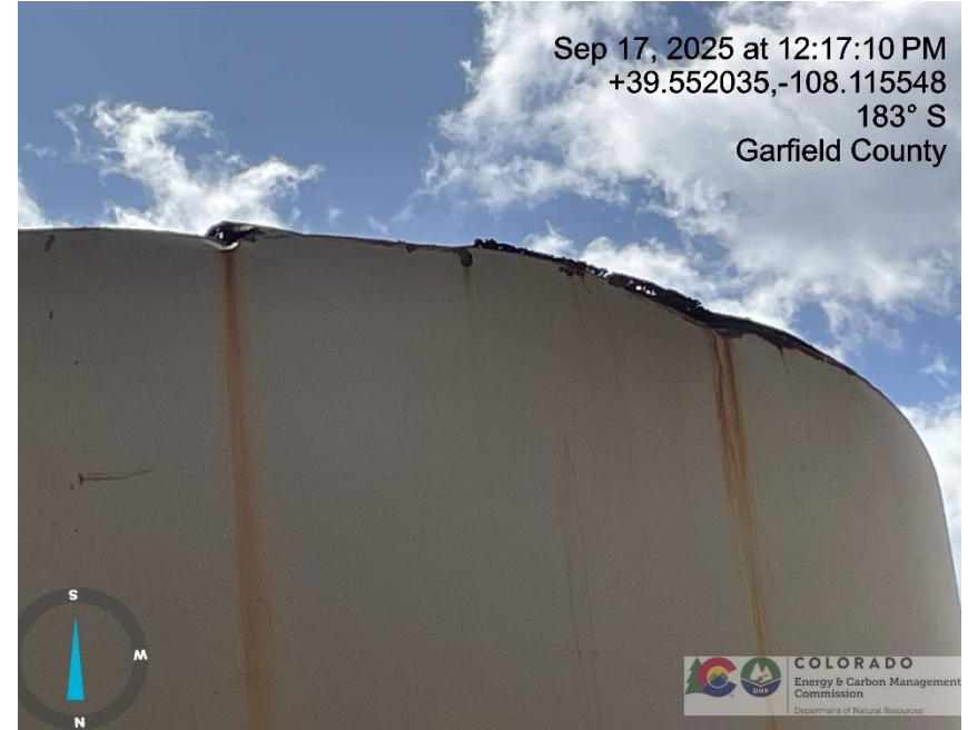
Photo # 276 Tank failure/tank lacks integrity
