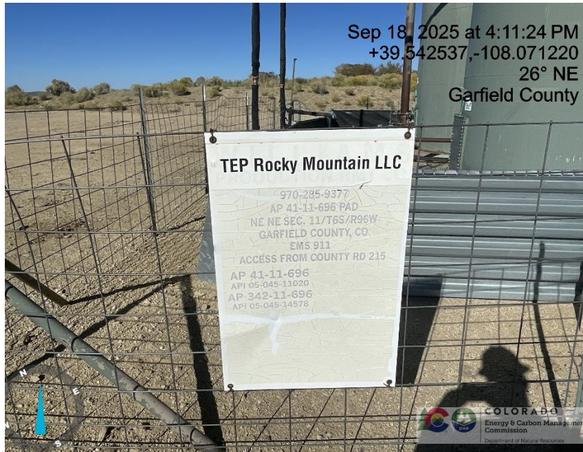
Photo # 1213 Battery sign weathered & faded/starting to become illegible
