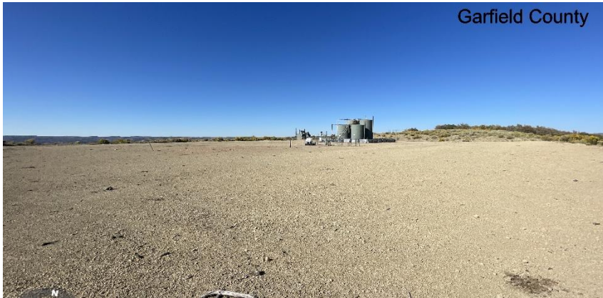
South West corner of location.
