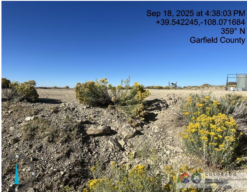
Photo # 1220 Erosion & transport of sediment off location /insufficient BMP's
