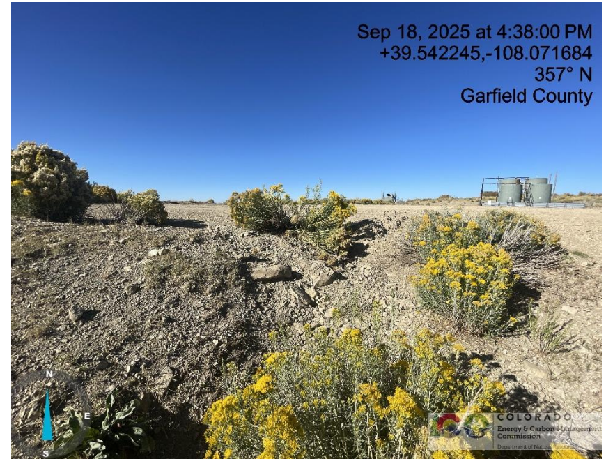
Photo # 1219 Erosion & transport of sediment off location /insufficient BMP's
