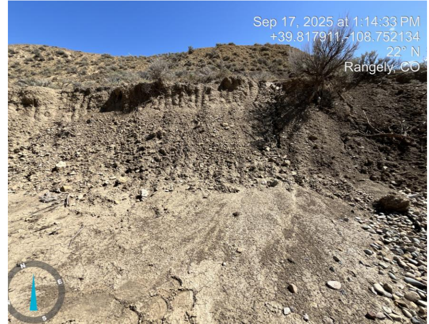
Photo # 3542 Erosion & transport of sediment on cutslope/sediment migrating onto location/insufficient BMP's
