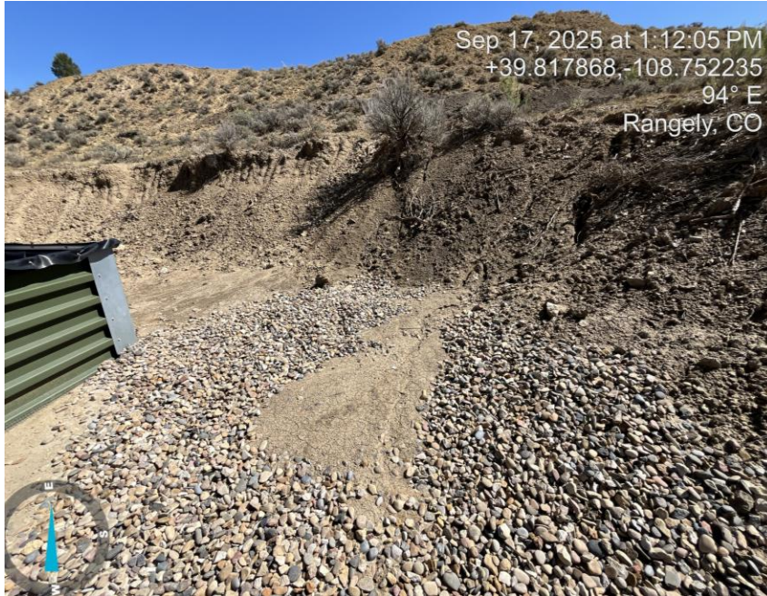
Photo # 3541 Erosion & transport of sediment on cutslope/sediment migrating onto location/insufficient BMP's
