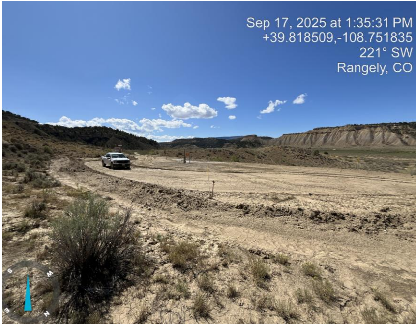
Photo # 3558 NE corner of location
