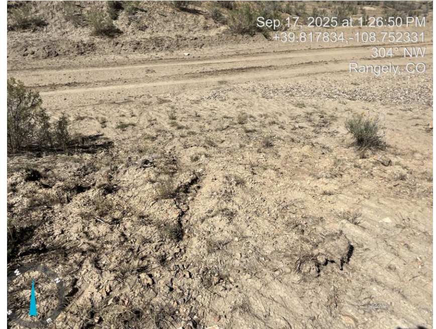
Photo # 3551 Failure to minimize erosion & transport of sediment
