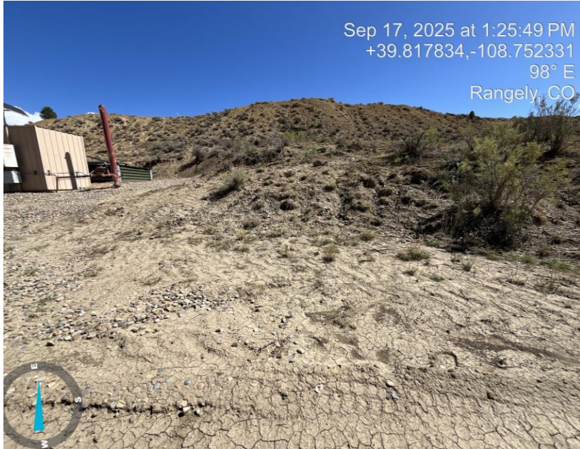
Photo # 3549 Failure to minimize erosion & transport of sediment
