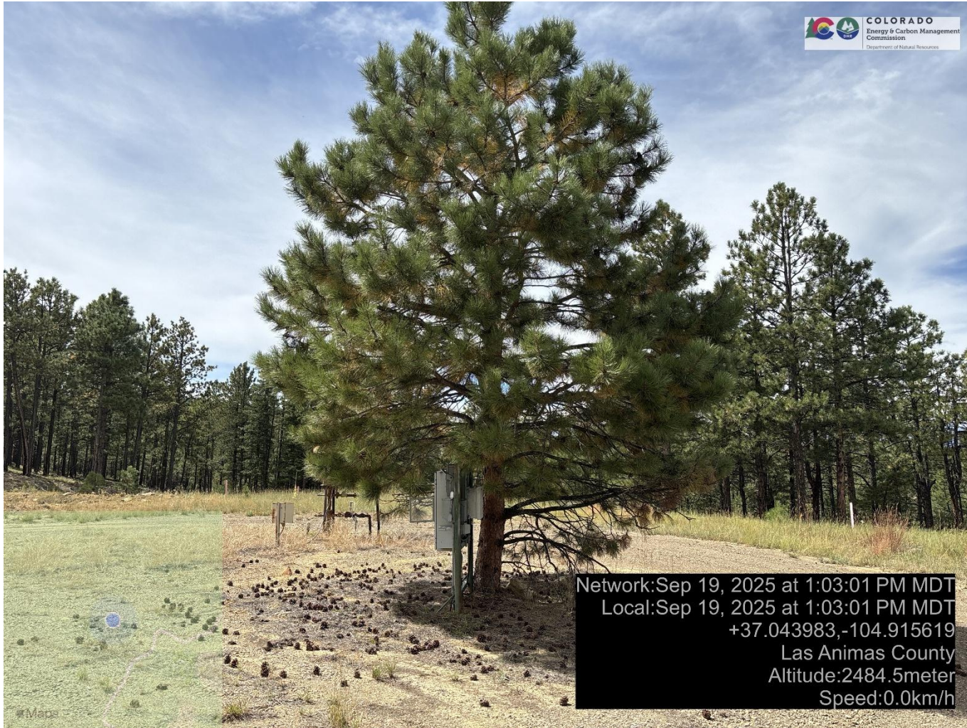
PHOTO 3: TREE GROWING OVER THE TOP OF ELECTRICAL PANEL AND VEGETATION AROUND WELLHEAD AND METER HOUSE. REMOVE TREE ON LOCATION AND MAINTAIN WEEDS AROUND ALL EQUIPMENT ON LOCATION PER RULE 606. CA DATE 10/19/2025.
