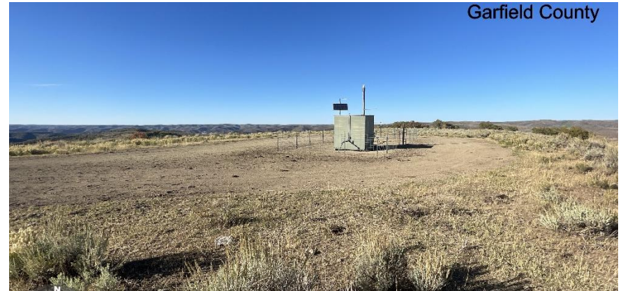
South East corner of location.
