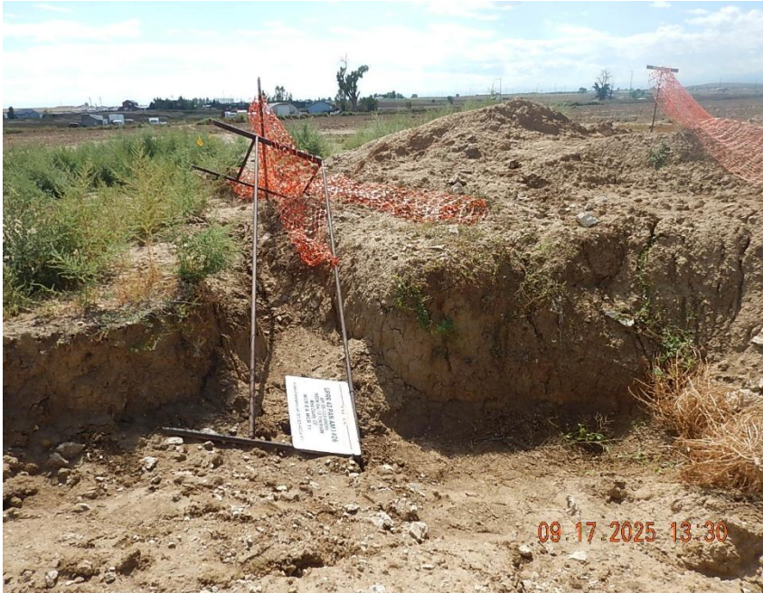
Signage at PA well; bottom of excavation
