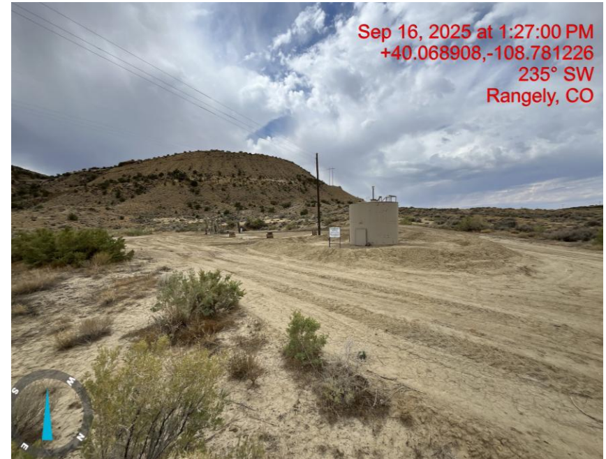
Photo # 3500 NE corner of location
