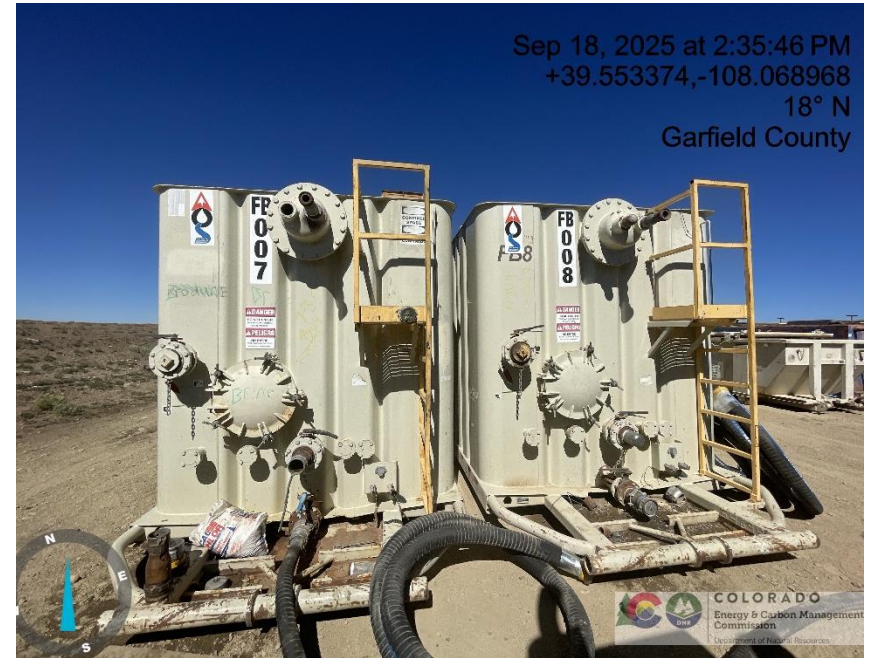
Photo # 1155 Frac tanks lack required labeling
