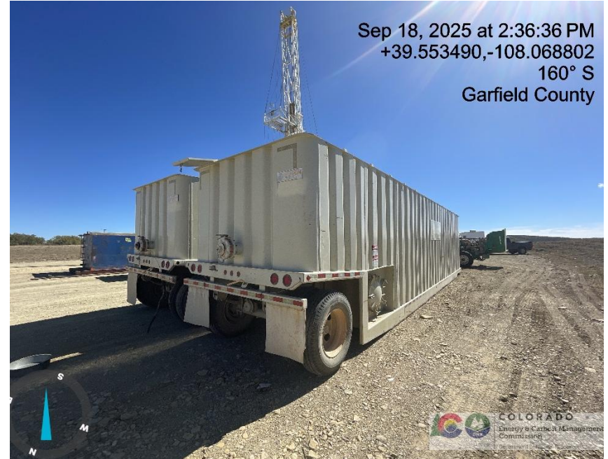
Photo # 1157 Frac tanks lack required labeling
