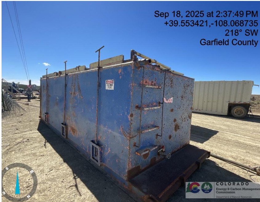
Photo # 1162 Rig tank lacks required labeling
