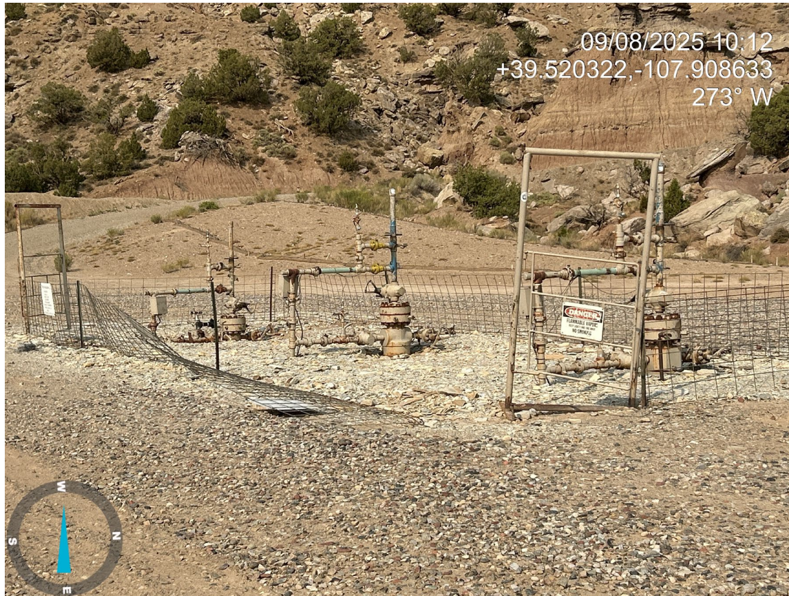
Photo 5: Photos showing fencing around the wellheads is in disrepair and insufficient to prevent livestock or wildlife entry. Maintenance is advised.
