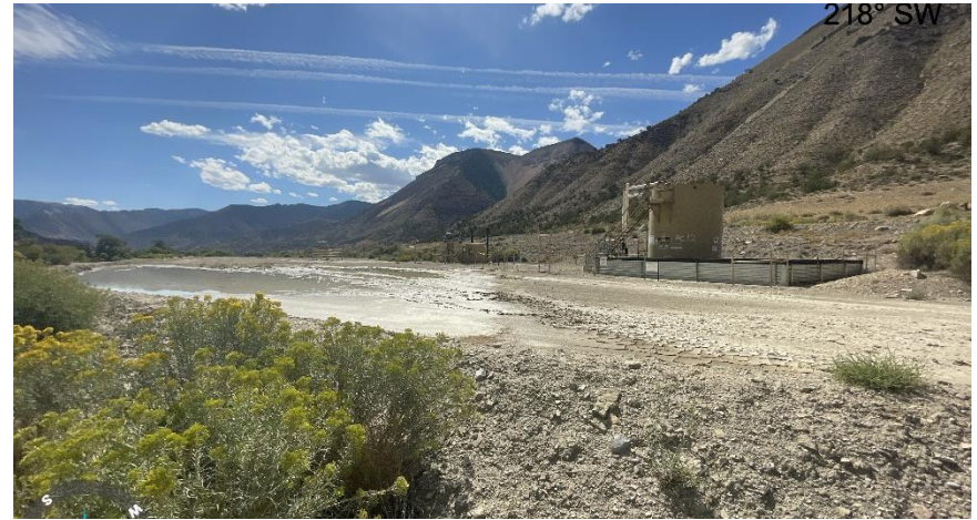
North East corner of location.
