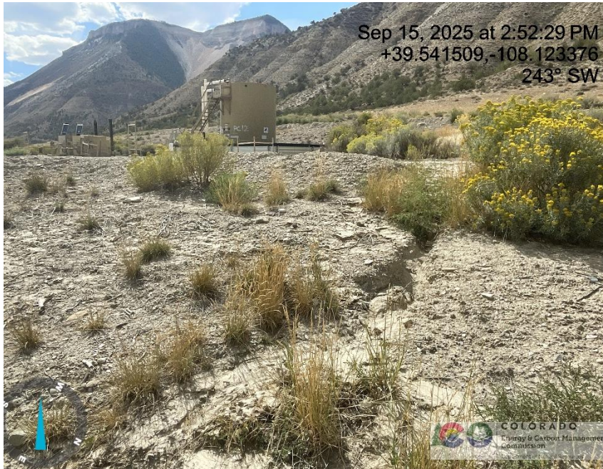
Photo # 9400 Erosion & transport of sediment off lease road & into a vegetated area/insufficient BMP's
