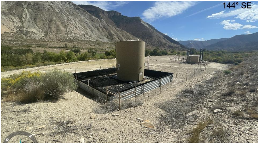
North West corner of location.
