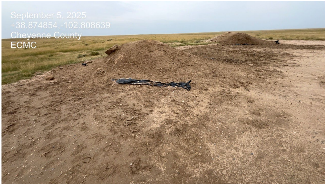
Photo 5. Facing toward southeast side of the location. The excavated impacted material was placed on a piece of plastic with no containment and some of the material has fallen outside of the liner. The plastic was also torn and compromised.
