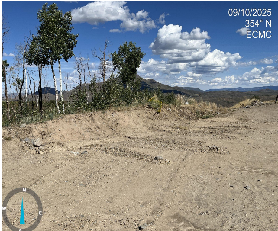
Photo 8. Photo taken on the western portion of the pad, facing north. Photo illustrates that the rock/debris pile has been removed.
