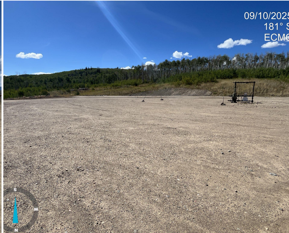
Photo 9. Photo taken near the entrance of the Location, facing south. Photo illustrates overview of Location. Additional trash/equipment has been removed.
