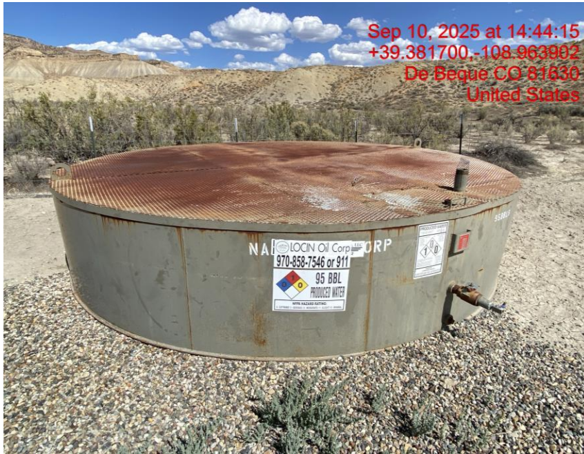
Location/No Secondary Containment for AST – Photo #00679
