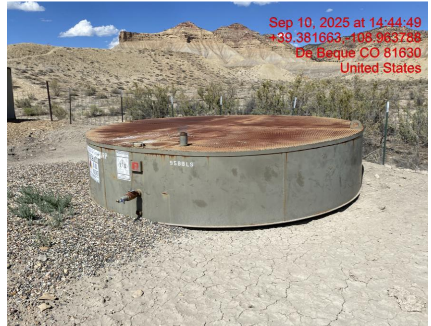
Location/No Secondary Containment for AST – Photo #00680
