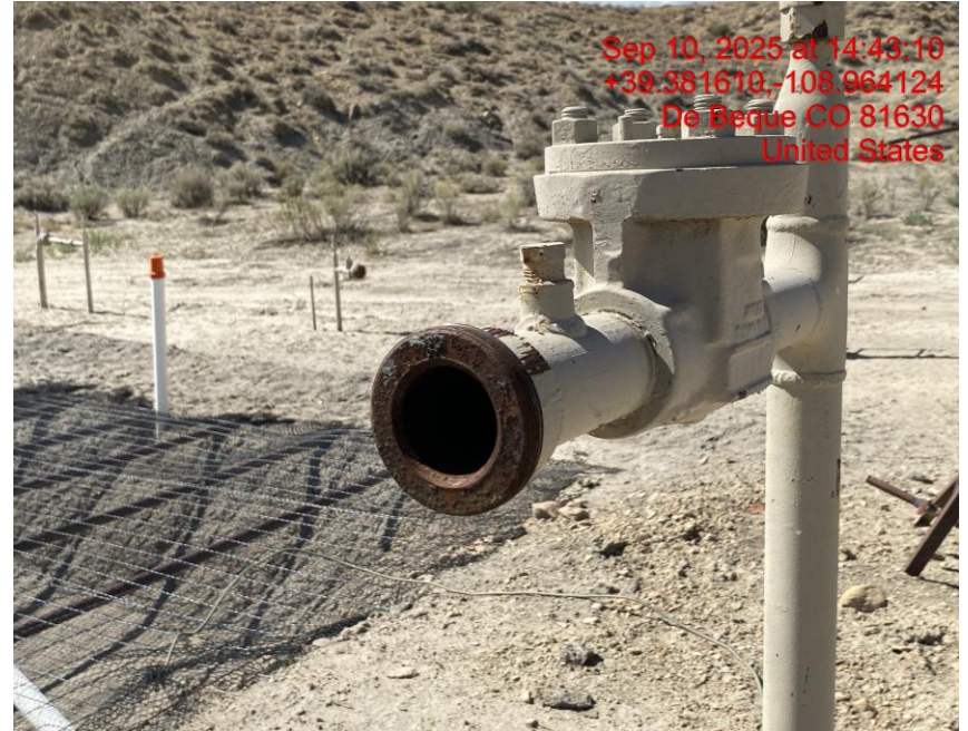
Open-Ended Flowline – Photo #00674
