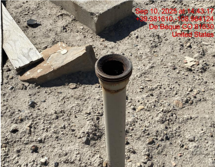
Open-Ended Flowline – Photo #00675
