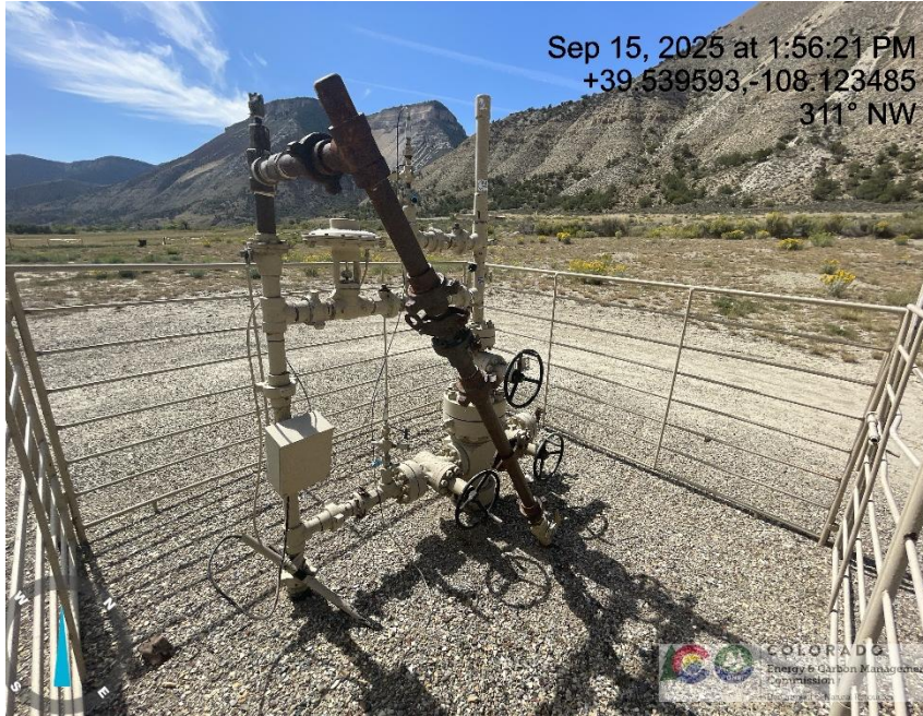
Photo # 9233 Bradenhead line tied into flowline/no FORM 4 SUNDRY
