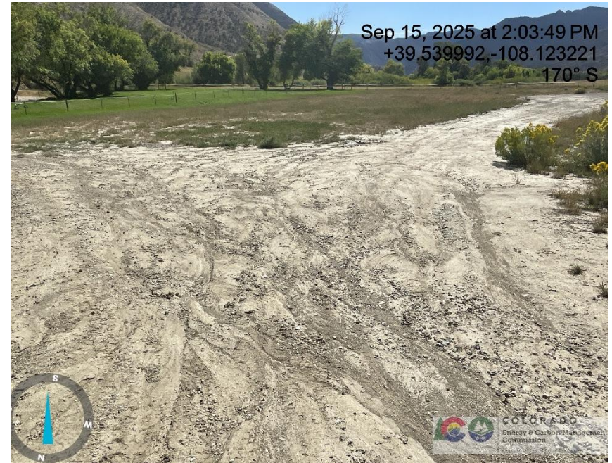
Photo # 9236 Erosion & transport of sediment on lease road & into a vegetated area/insufficient BMP's
