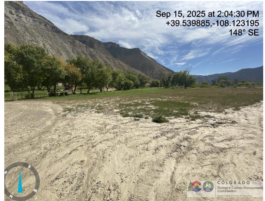
Photo # 9238 Erosion & transport of sediment on lease road & into a vegetated area/insufficient BMP's
