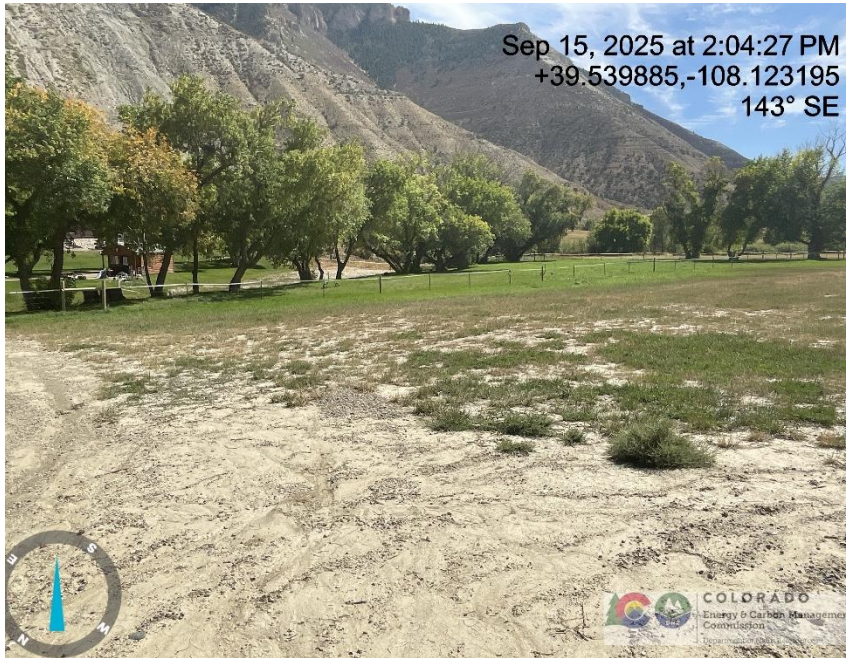
Photo # 9239 Erosion & transport of sediment on lease road & into a vegetated area/insufficient BMP's
