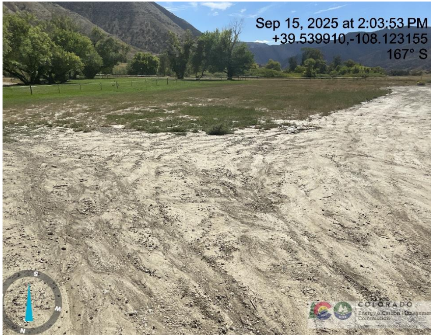
Photo # 9237 Erosion & transport of sediment on lease road & into a vegetated area/insufficient BMP's
