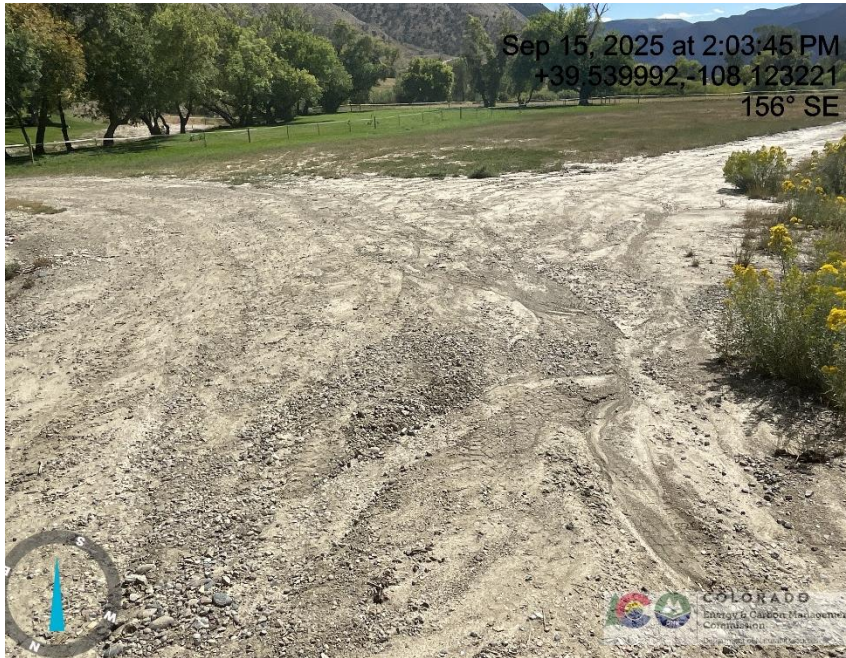
Photo # 9235 Erosion & transport of sediment on lease road & into a vegetated area/insufficient BMP's
