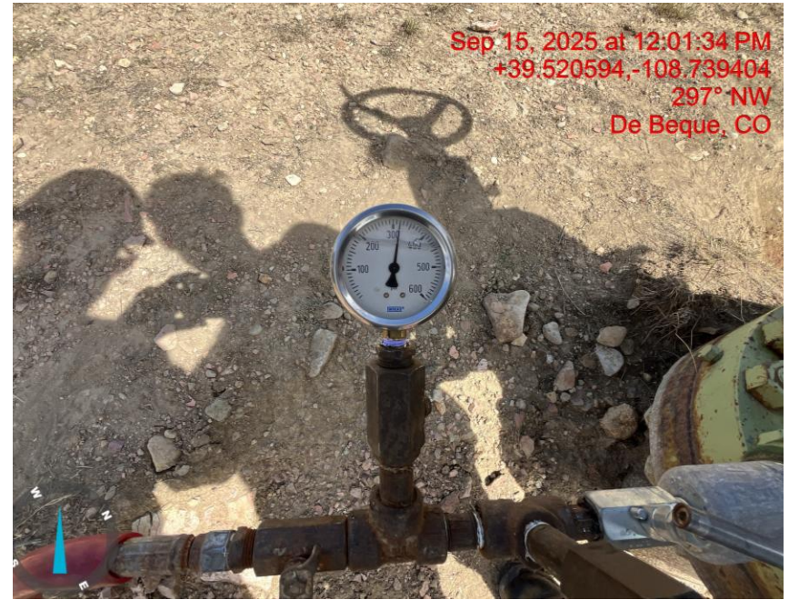
Photo # 3426 Final test pressure
