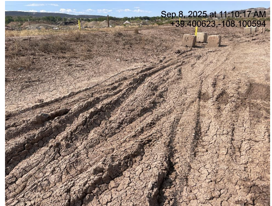
Photo # 6383 Lack of stabilization/compaction on location
