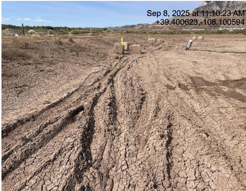
Photo # 6382 Lack of stabilization/compaction on location
