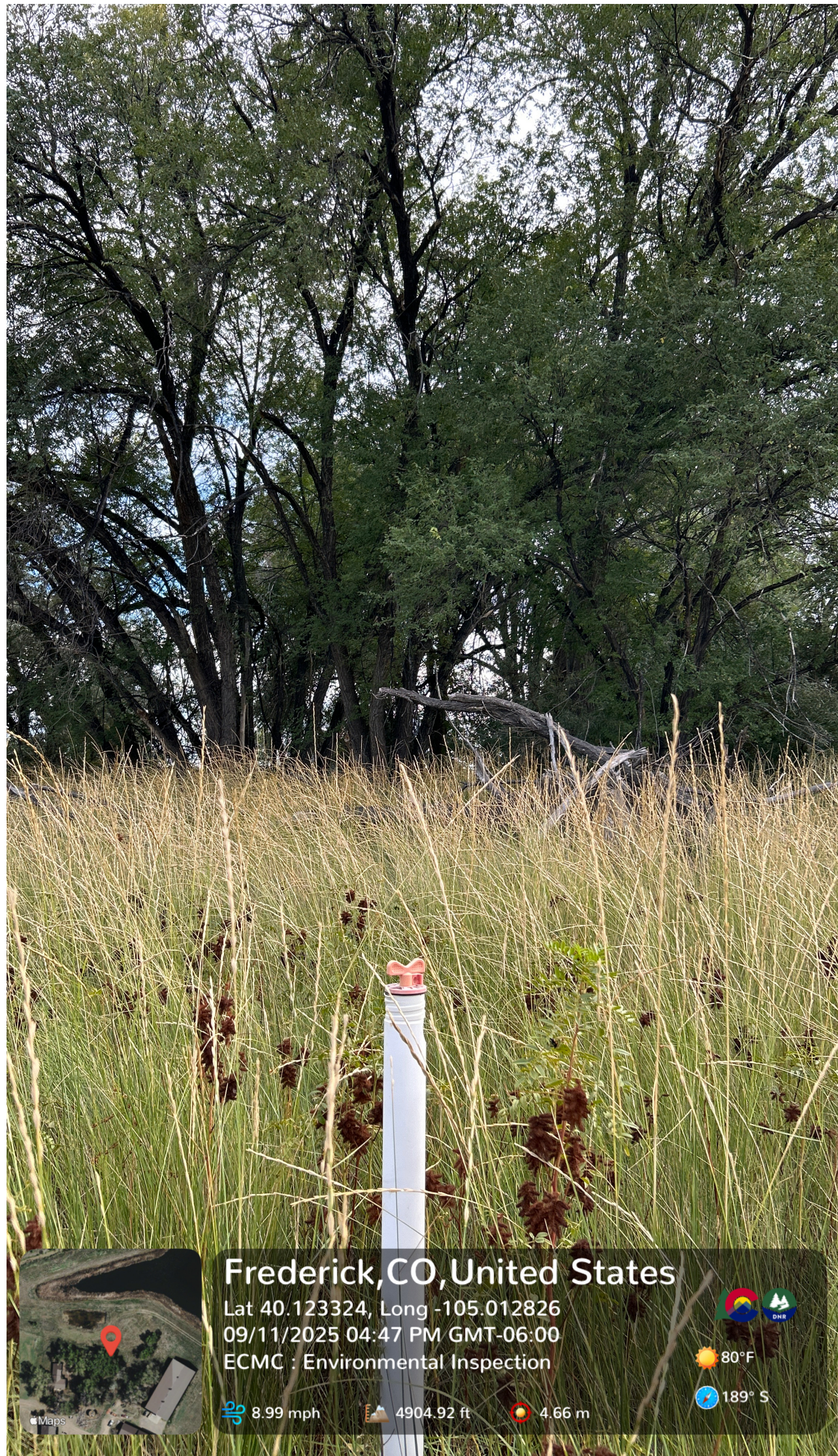
A network of monitoring wells completed as stickups was visible on location.
