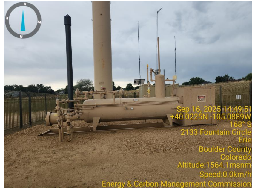
Photo 6 Horizontal Heated Separator & ECD.
