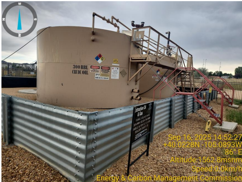
Photo 5 Tank battery.
