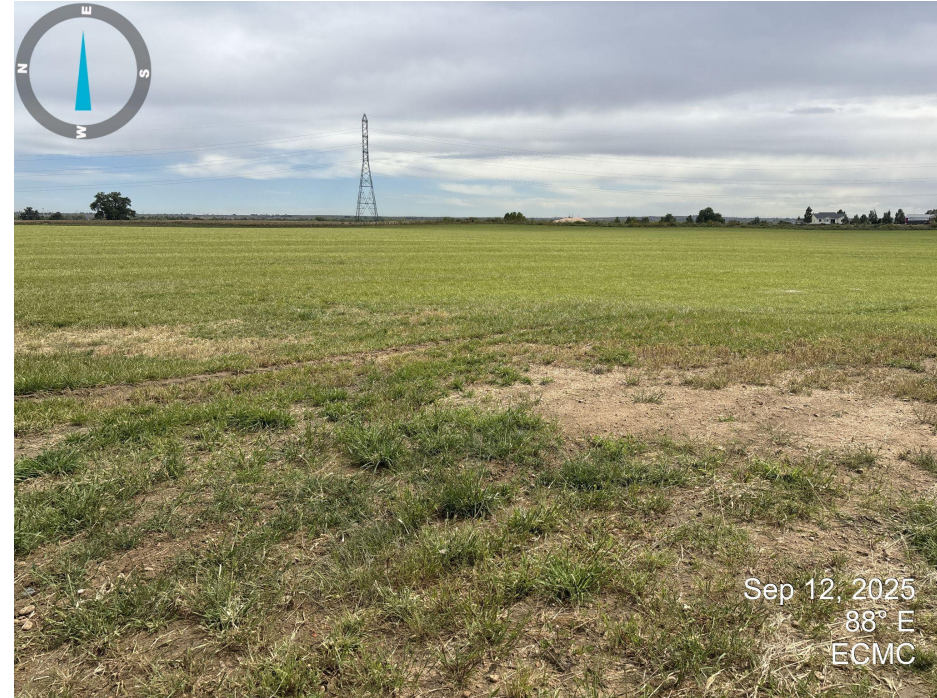
Photo 6. Looking east from the wellhead area. All oil and gas equipment has been removed from this area. The area has not yet been returned to cropland or recontoured.
