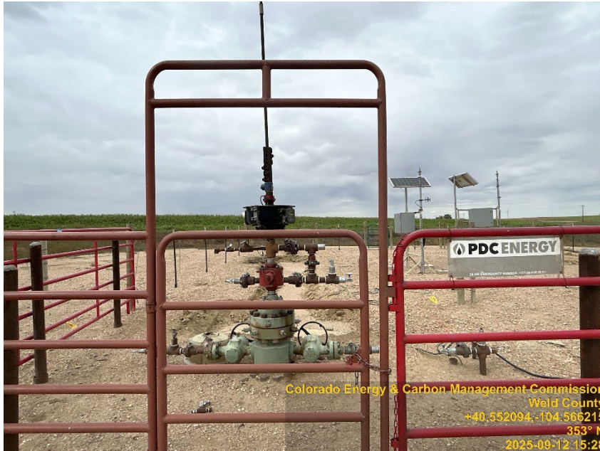
Photo #3 Dillard 20T-221 (123-36602) Wellsite Temporarily Abandoned | TA Pumpjack(s) removed
