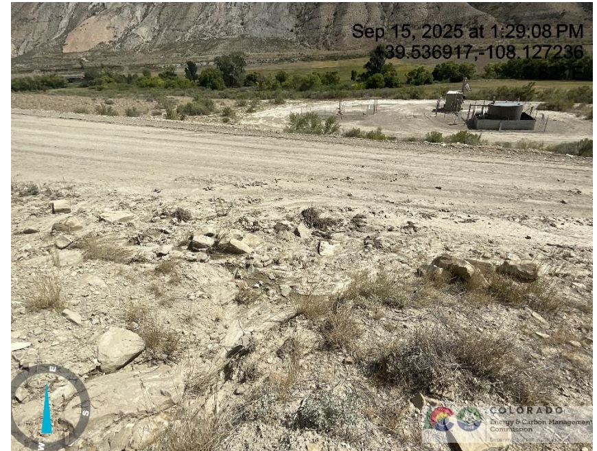
Photo # 8562 Erosion & transport of sediment onto lease road/insufficient BMP's (approximately 5/10th of a mile from entrance to location)
