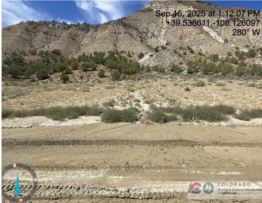
Photo # 8533 Erosion & transport of sediment onto lease road/insufficient BMP's (approximately 3/10th of a mile from entrance to location)
