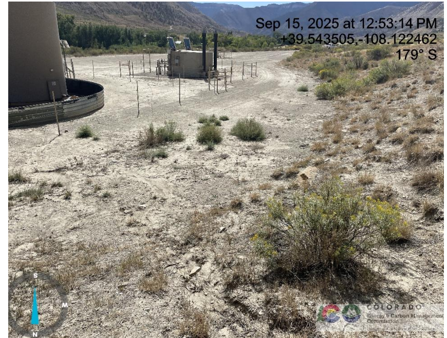
Photo # 8520 Erosion & transport of sediment onto location /insufficient BMP's
