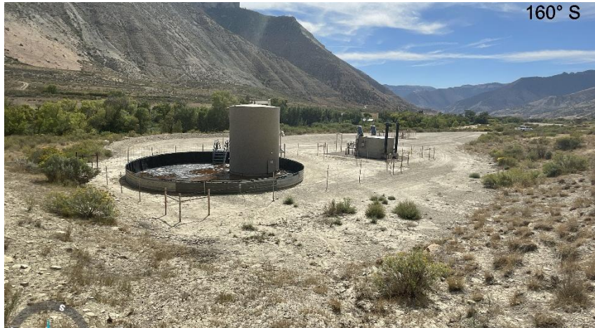
North West corner of location.
