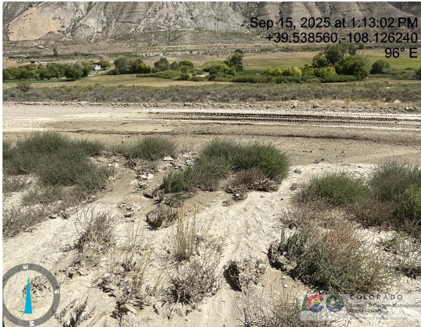
Photo # 8535 Erosion & transport of sediment onto lease road/insufficient BMP's (approximately 3/10th of a mile from entrance to location)
