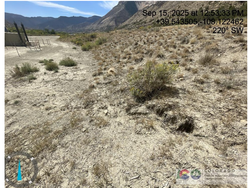
Photo # 8516 Erosion & transport of sediment onto location /insufficient BMP's
