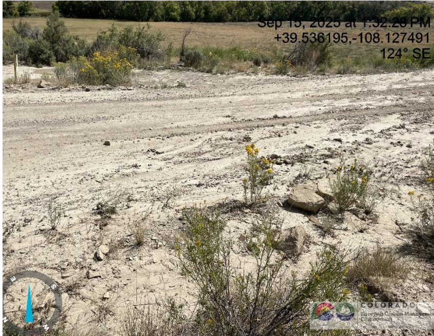
Photo # 8567 Erosion & transport of sediment onto lease road/insufficient BMP's (approximately 6/10th of a mile from entrance to location)
