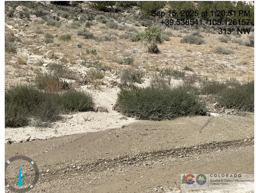
Photo # 8544 Erosion & transport of sediment onto lease road/insufficient BMP's (approximately 3/10th of a mile from entrance to location)
