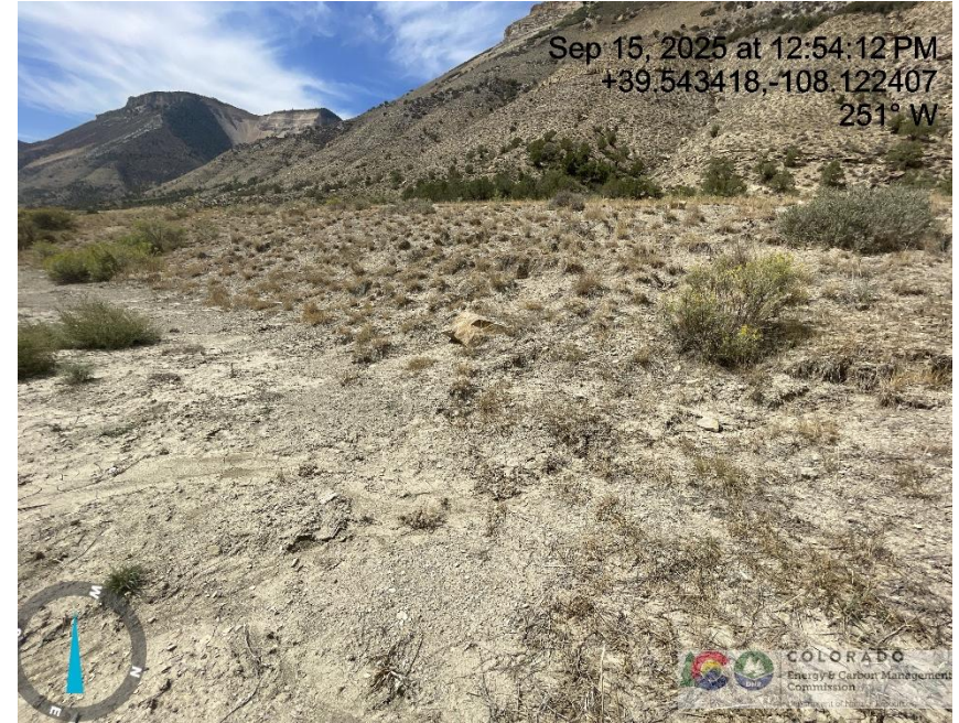
Photo # 8518 Erosion & transport of sediment onto location /insufficient BMP's
