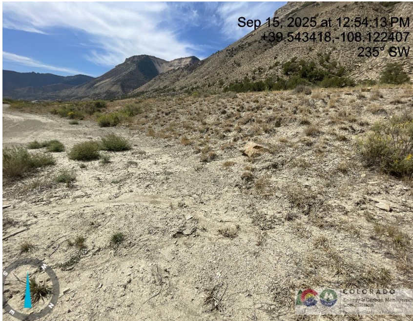
Photo # 8519 Erosion & transport of sediment onto location /insufficient BMP's
