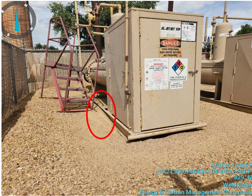
Photo 11: Equipment not anchored
