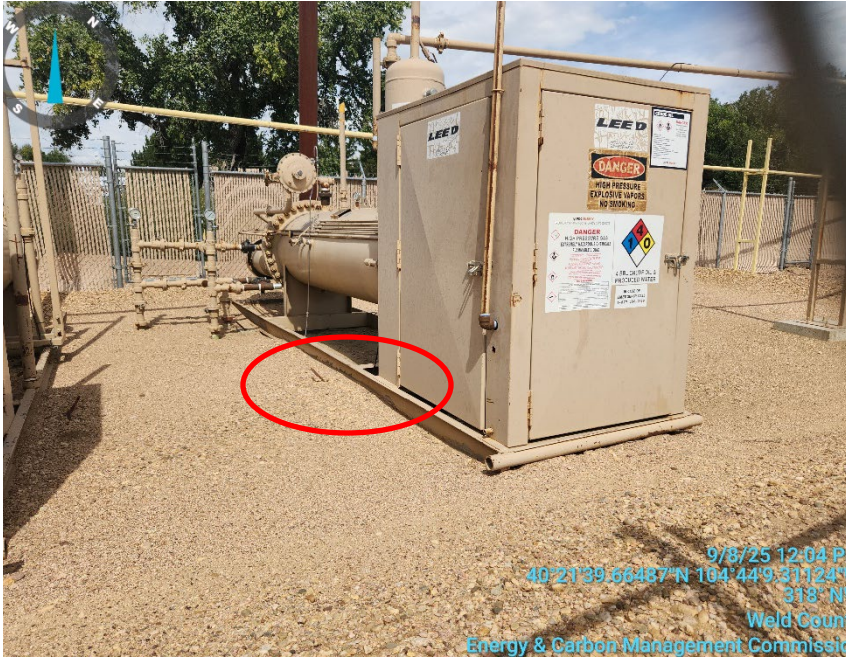
Photo 9: equipment not anchored
