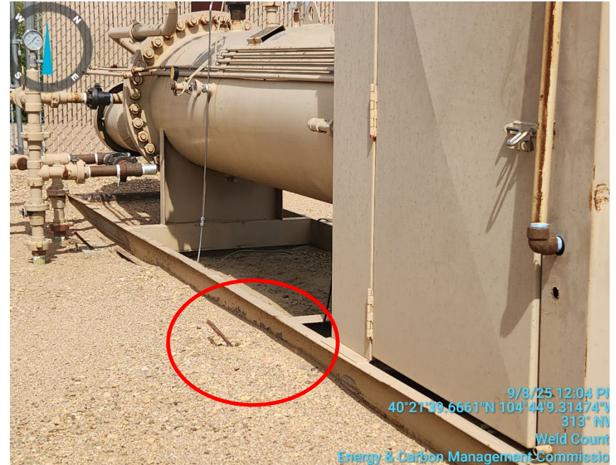
Photo 10: equipment not anchored
